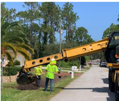
Swale Grading Emerson
