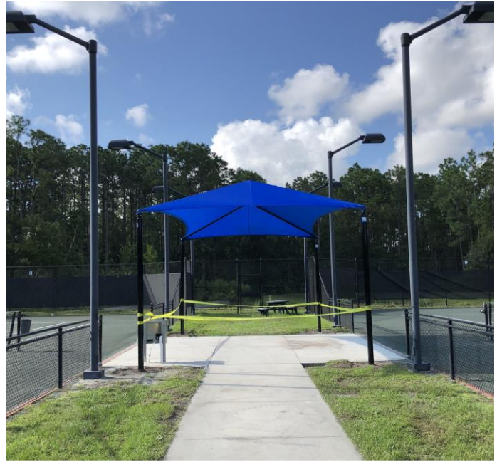
Tennis Center Shade Canopy
