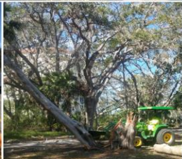
Removing hazardous trees St Joe's walkway
