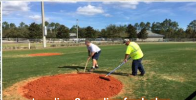
Leveling & grading fresh clay ITSC
