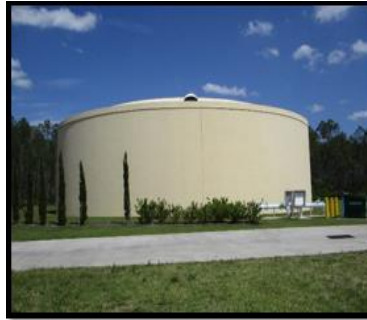
2 million gallon storage tank
