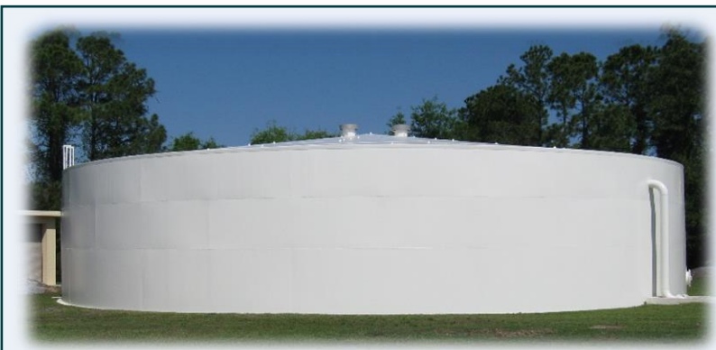
6 Water Storage Tanks Capacity of 7.5 Million Gallons
