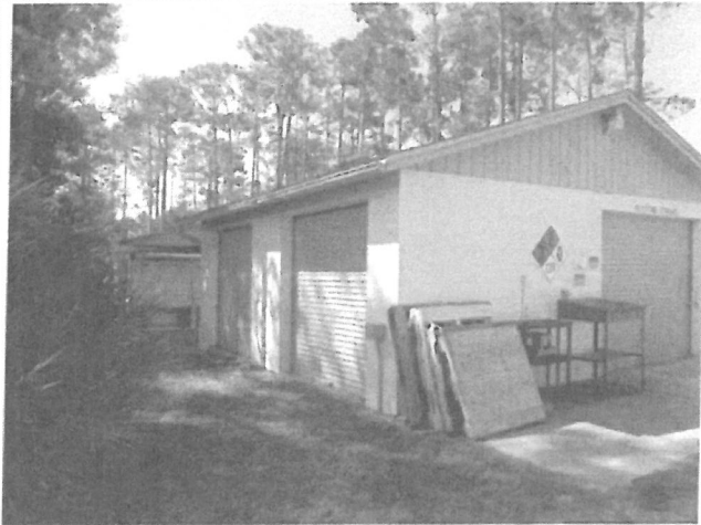
Pesticide Storage Building
