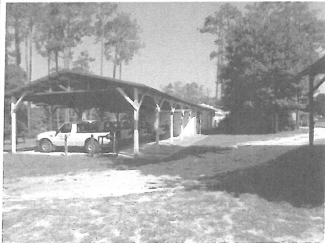
Additional Equipment Storage Barn
