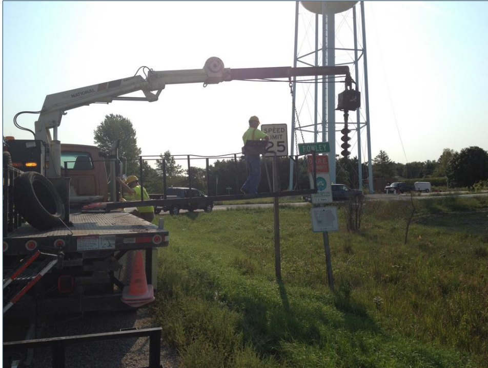
Figure 3-13: Installation of LED speed limit sign
