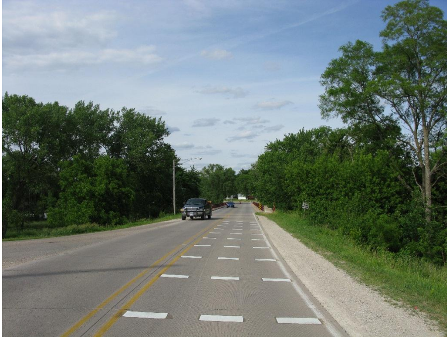
Figure 5-11: Transverse bar treatment at south Quasqueton entrance
