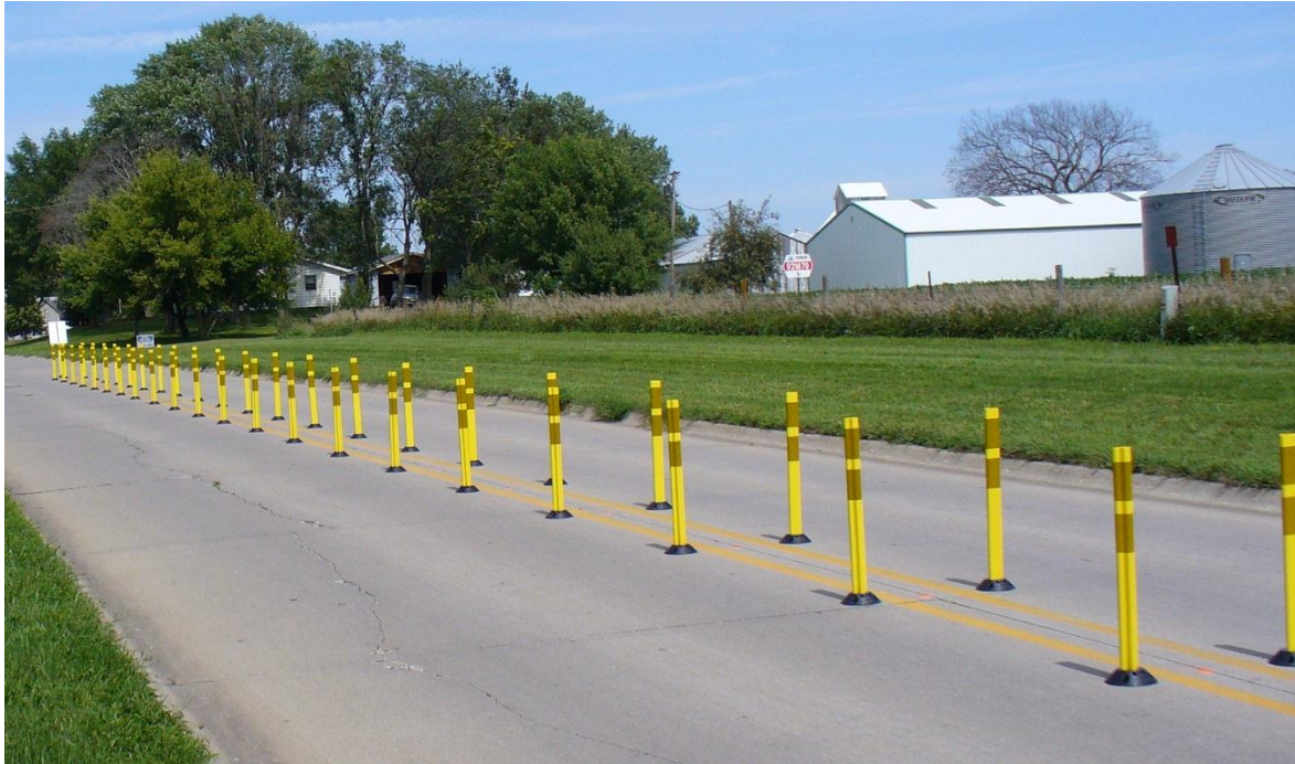
Figure 3-9: Temporary island treatment in Slater, Iowa
