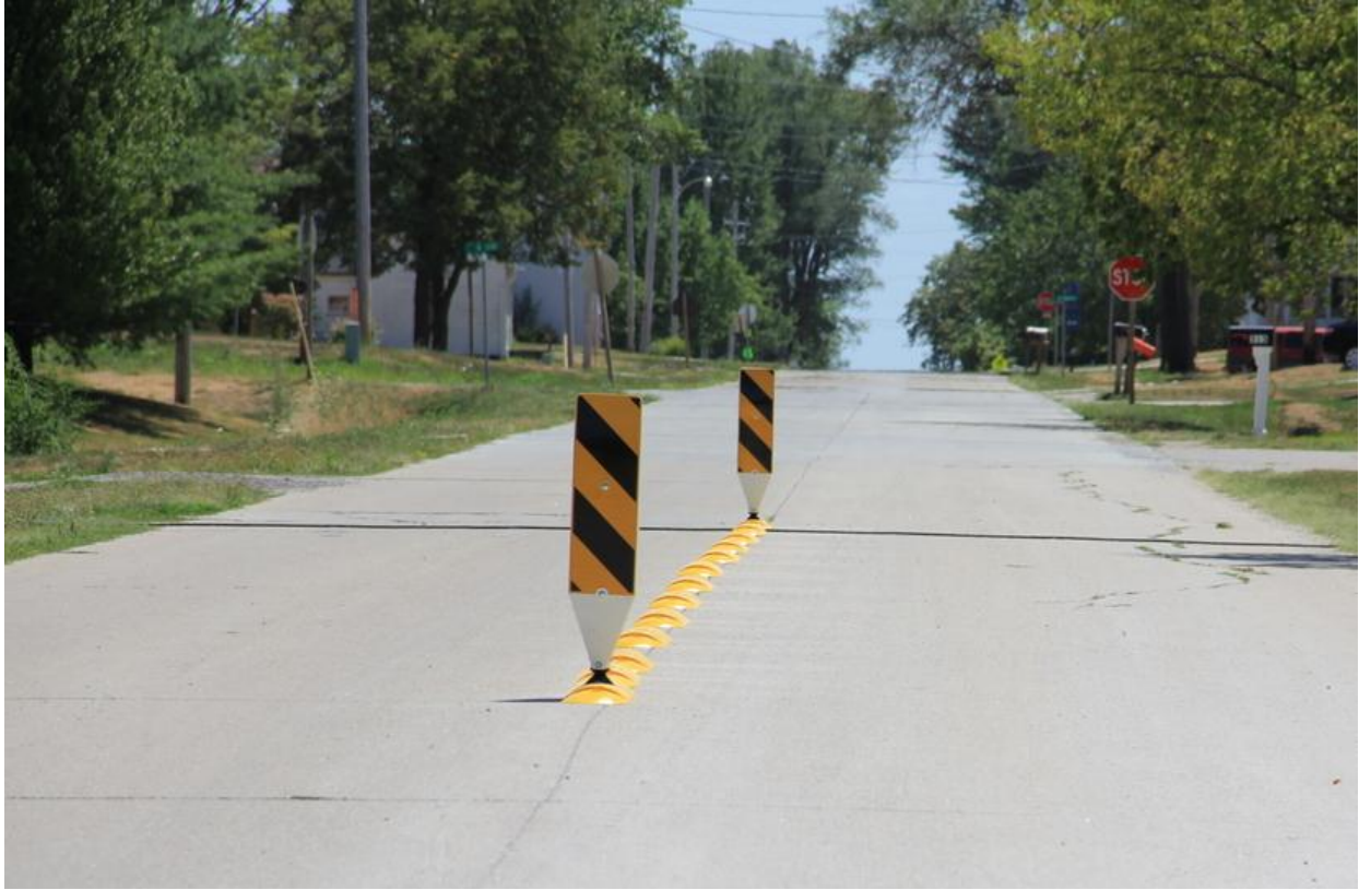
Figure 3-10: Raised median with hazard markers at each end
