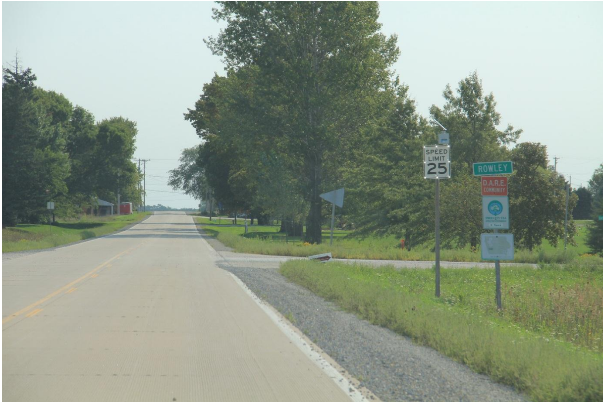
Figure 5-18: Radar-activated LED speed limit sign installed at west Rowley community entrance
