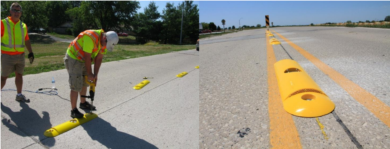
Figure 3-11: Installation of raised curbing (left) and close-up of raised curbing (right)
