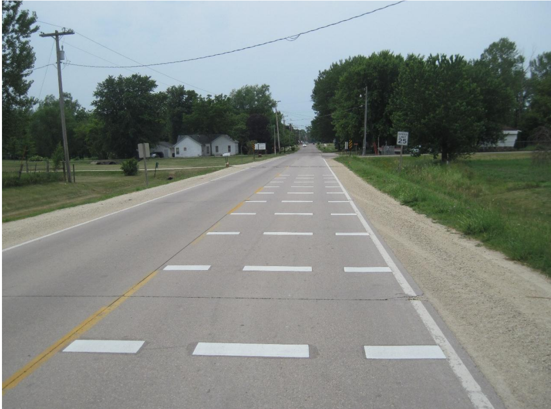
Figure 5-2: Transverse bar treatment at Hazleton east entrance
