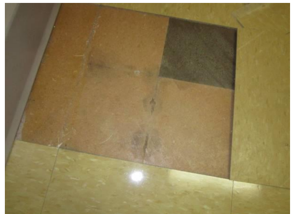
Photo #24 Visible mold and musty odor between floor tile layers in east hallway by Room 156.
