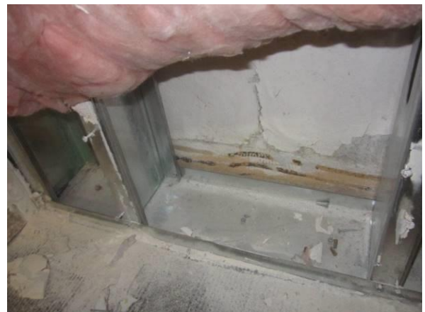
Photo #18 Concrete wall behind recently built-out gypsum wall at base of southeast wall in Room 129.
