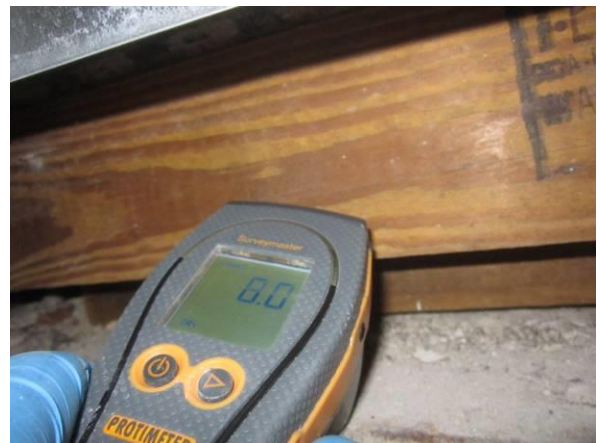
Photo #6 Dry moisture measurement in old wood in southwest upper wall cavity of Evidence Storage.
