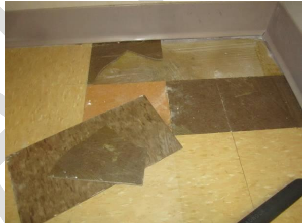
Photo #22 Visible mold below bottom floor tile layer by drinking fountain in west hallway by restrooms.
