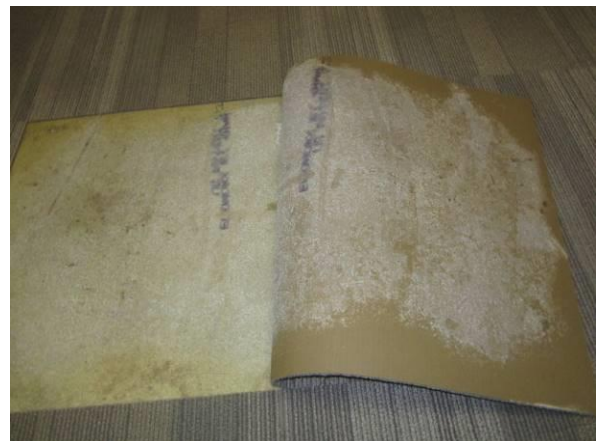
Photo #30 Wet carpet glue below carpet square in IT Room 150.
