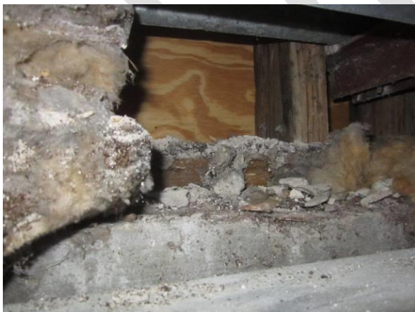
Photo #17 Bat guano at top of concrete wall in southeast corner of Room 129.
