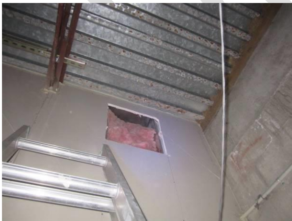
Photo #11 Upper wall cut at southwest corner of Room 129.
