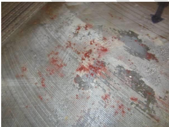
Photo #23 Wet glue, red staining and musty odor below carpet square in Room 165.
