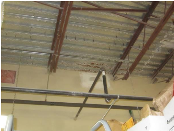
Photo #3 Corrosion on metal roof deck within the southwest portion of the evidence storage room.
