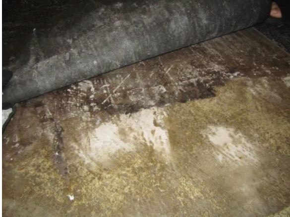
Photo #19 Visible mold below carpet square by entrance to the Sheriff's Office Room 178.
