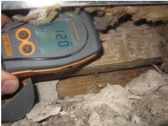
Photo #13 Dry moisture measurement in old wood on upper southwest wall in Room 129.
