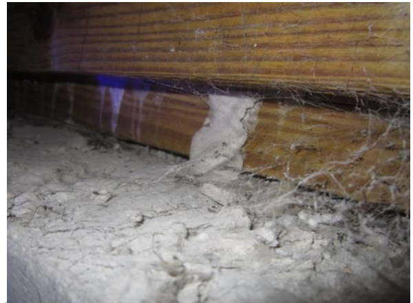
Photo #14 View of old wood on upper south center wall in Room 129.
