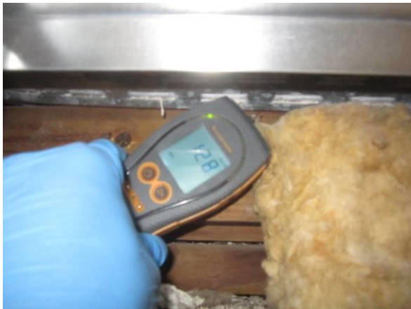
Photo #9 Dry moisture measurement on old wood on upper wall in Narcotics Storage
