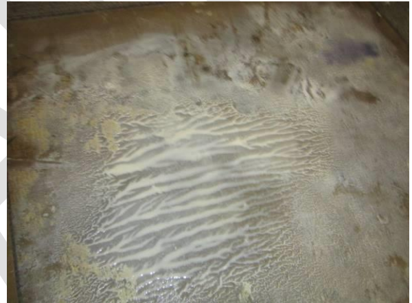
Photo #28 Close up of wet carpet glue in Room 103.
