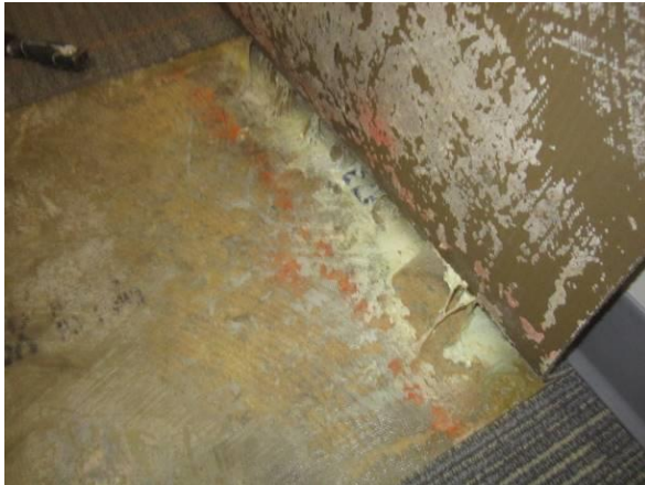
Photo #21 Moisture and mold below carpet square in Room 168.
