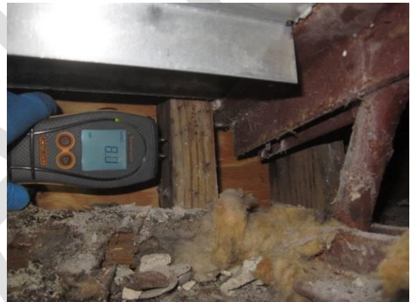
Photo #16 Dry moisture measurement in old wood by bat droppings at southwest corner of Room 129.
