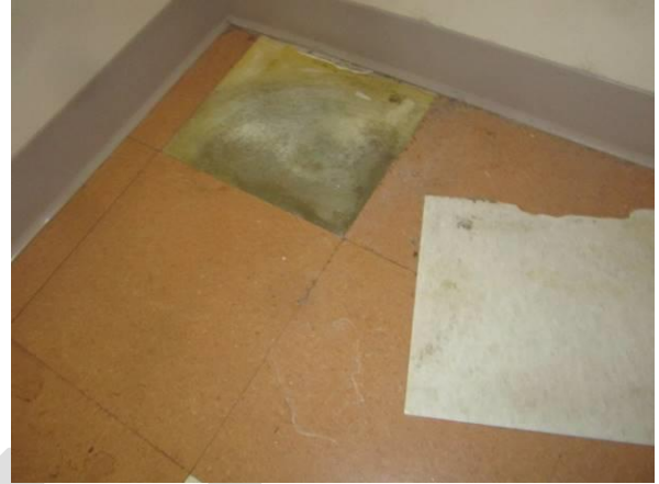
Photo #26 Mold below floor tile in Room 127.
