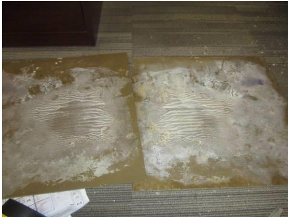
Photo #27 Wet carpet glue in Room 103.
