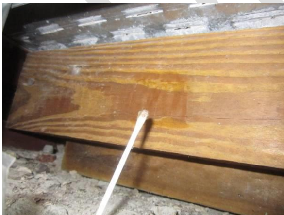
Photo #5 Swab testing on old wood in old wood in southwest upper wall cavity of Evidence Storage.
