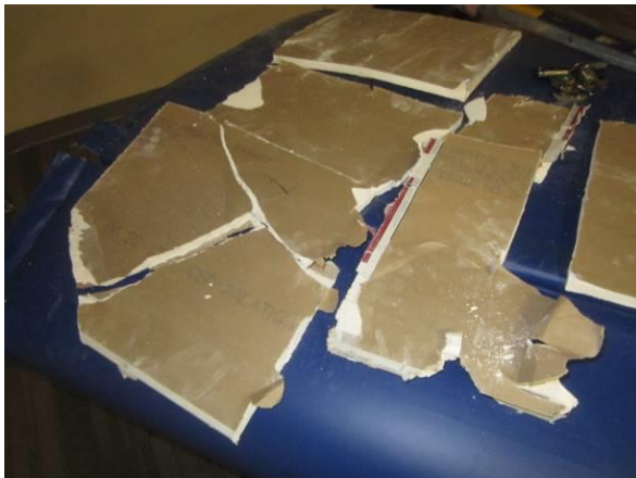
Photo #15 No visible mold growth on back of drywall at cut locations in Room 129.
