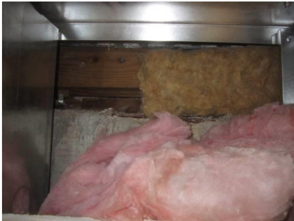
Photo #7 Old wood and insulation along upper south wall in Narcotics Storage.
