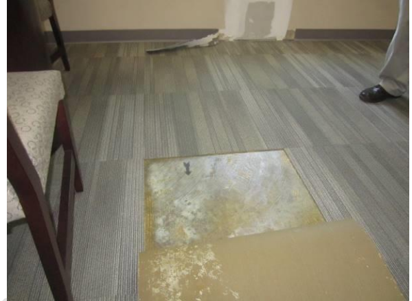
Photo #20 No moisture or mold issues identified below carpet square in Room 175.
