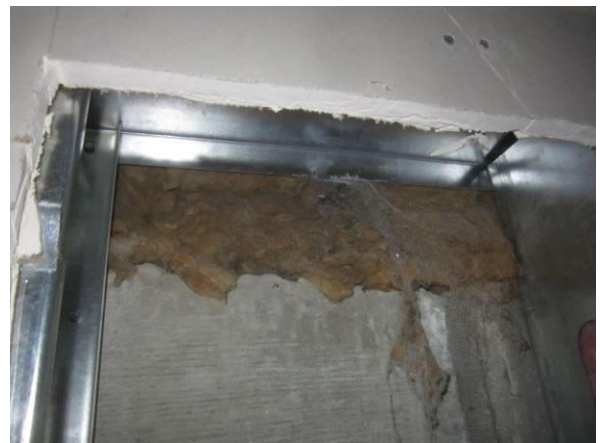
Photo #12 Old fiberglass on top of concrete upper wall in southwest corner of Room 129.
