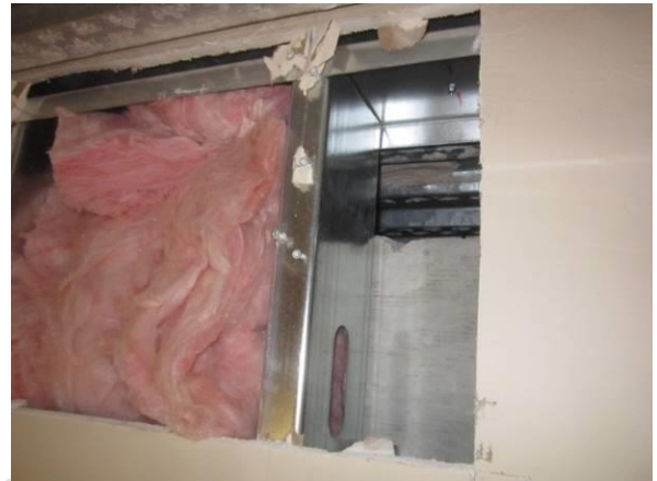
Photo #2 Typical view of new fiberglass and metal studs in upper wall cavity cuts in the southeast east portion of the evidence storage room.
