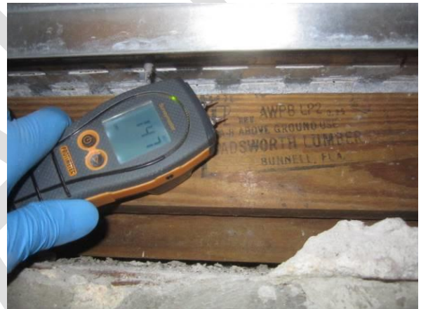
Photo #4 Dry moisture measurement in old wood framing blocking at top of concrete wall in southwest corner of the evidence storage room.
