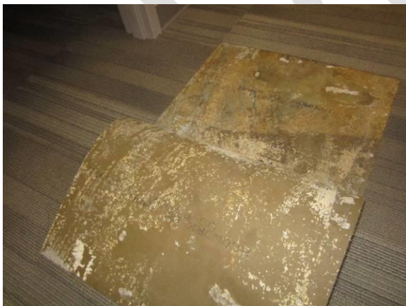
Photo #29 Musty odor and mold below carpet square in Room 105A.
