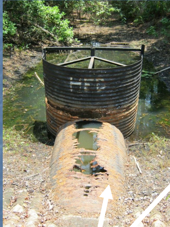
L-1 Structure Structural Rate = 6
