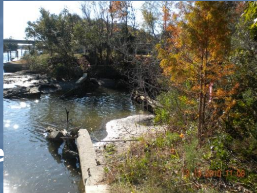
Emergency - Mulberry Creek Headwall Replacement Cost $251,000 April 2011
