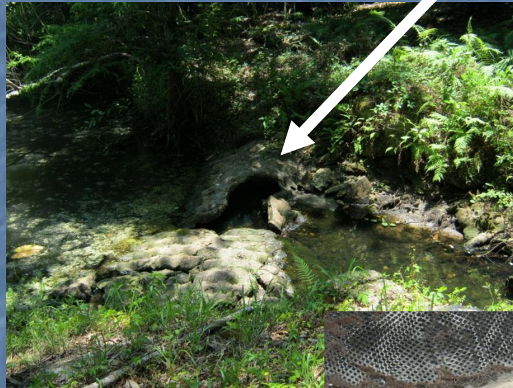
M-2 Structure Mulberry Creek Hazard Rating = 1
