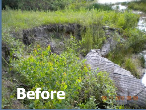
Emergency Rippling Waterway Structure Cost $85,000 July 2010
