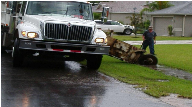
Past Swale Maintenance - Ditchmaster
