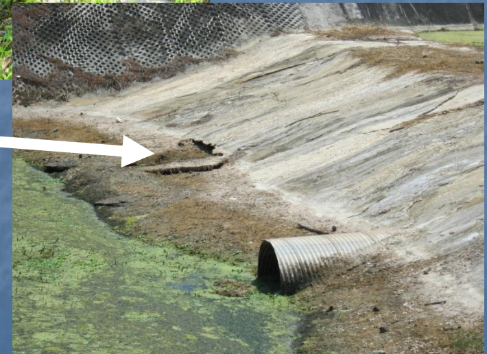
R-1 Structure Royal Palms Canal Hazard Rating = 6
