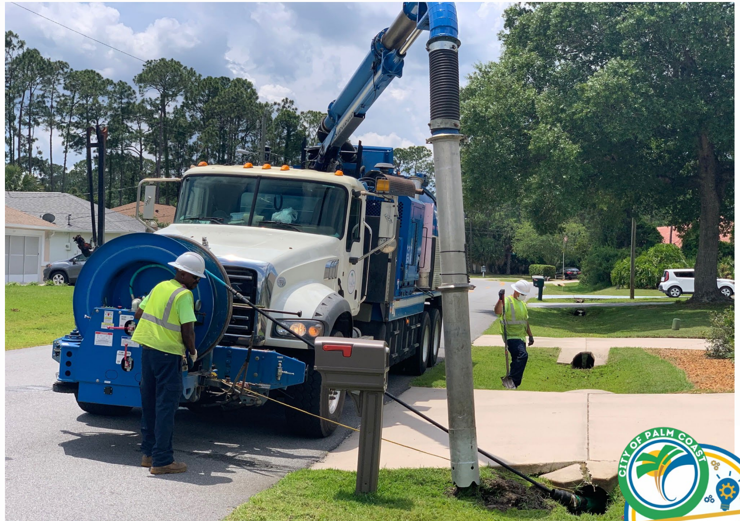
Two Culvert Crews
