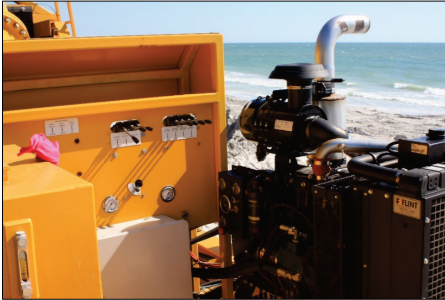
Figure 17. FRS diesel prime mover and hydraulic control station.
