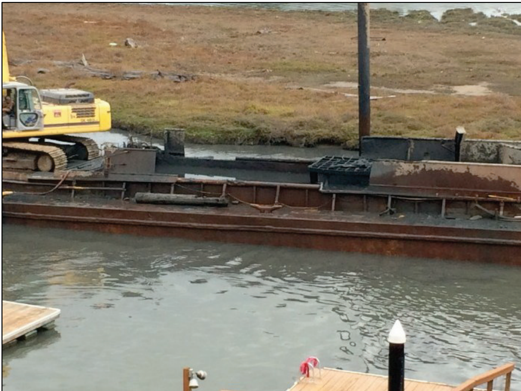
Figure 12. Small bottom-door barge with fixed grizzly – San Francisco Bay, CA.
