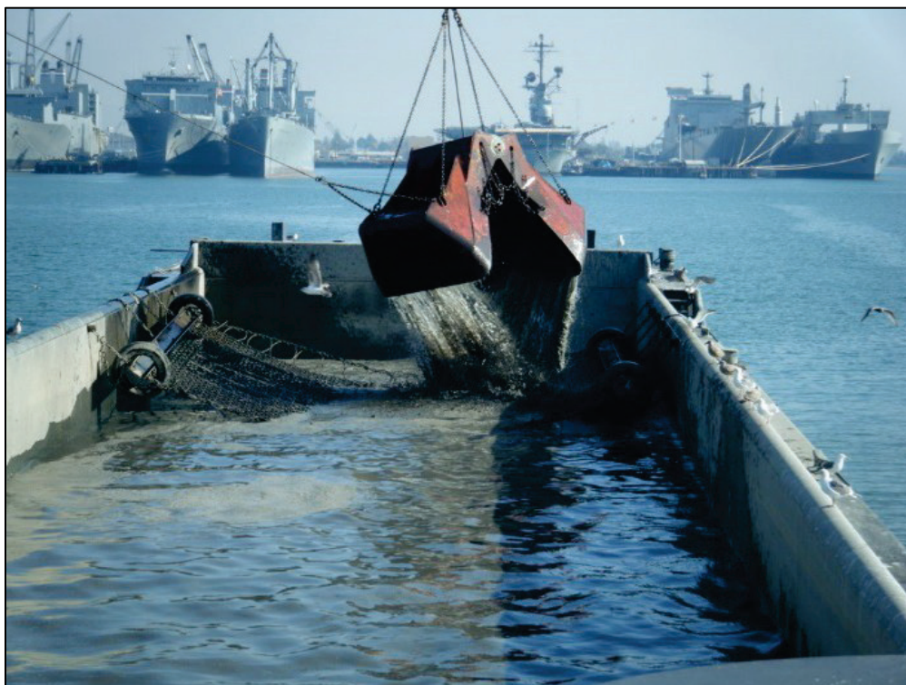
Figure 11. Barge screen constructed of chain used in a CA dredging project (Hoffman et al. 2015).
