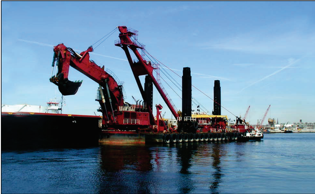
Figure 4. Mechanical (backhoe) dredge.
