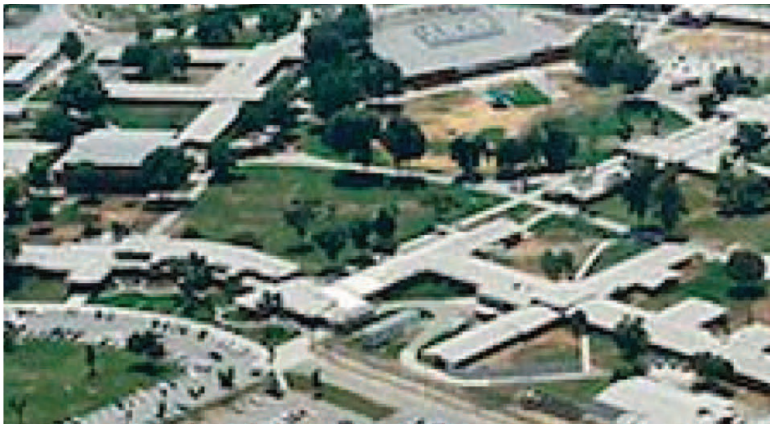
Photo courtesy of the California Department of Corrections and Rehabilitation
