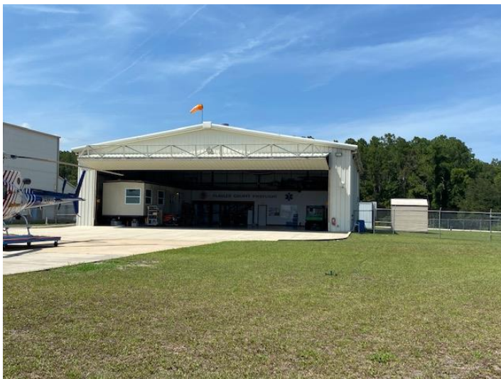
View of typical free standing Box Hangar
