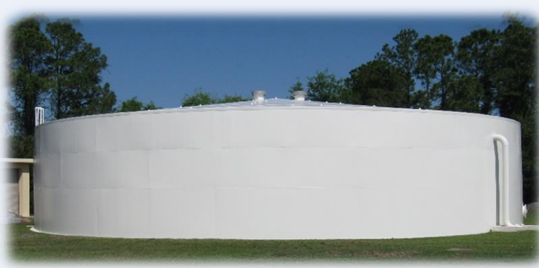
6 Water Storage Tanks Capacity of 7.5 Million Gallons
