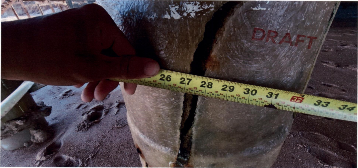
BENT 49 PILE F 5'x3" DEEP CRACK
