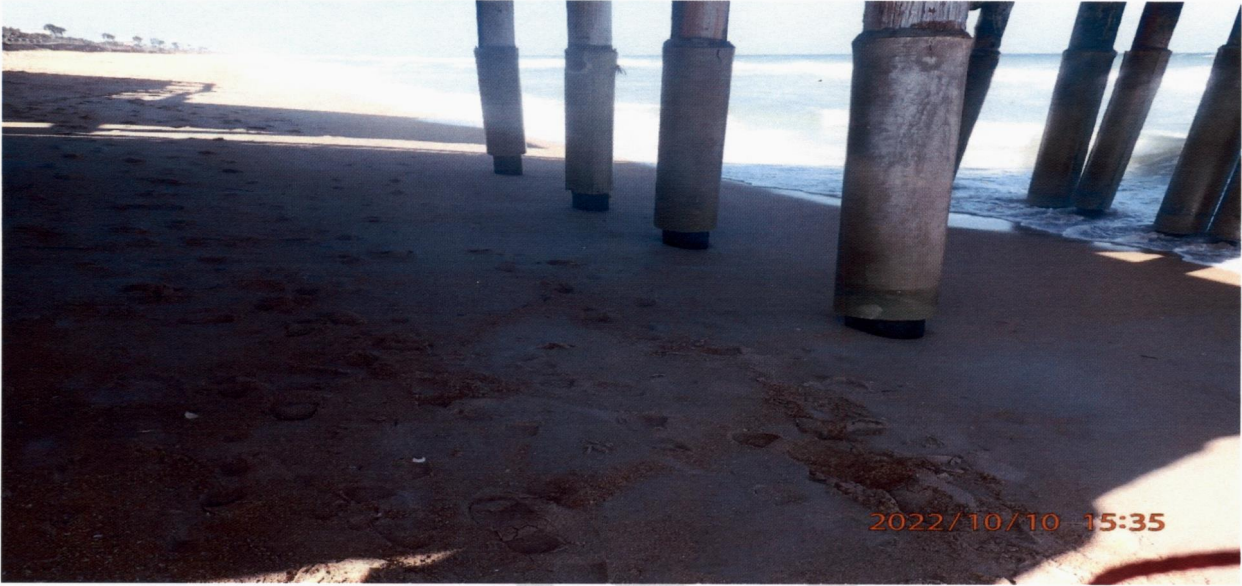
BENT 37 HORIZONTAL CROSS BRACE NO LONGER ATTACHED
