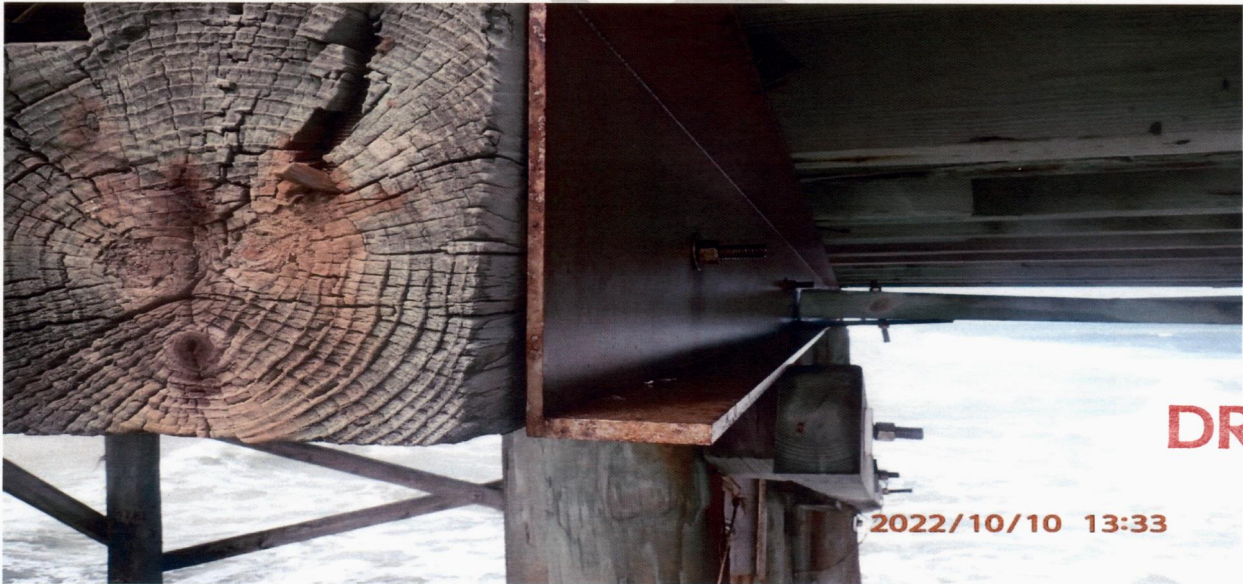
BENT 39 CAP REPAIR EASTSIDE
