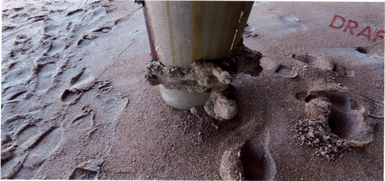
BENT 48 PILE J WITH STAINLESS STEEL CLAMP — TYPICAL
