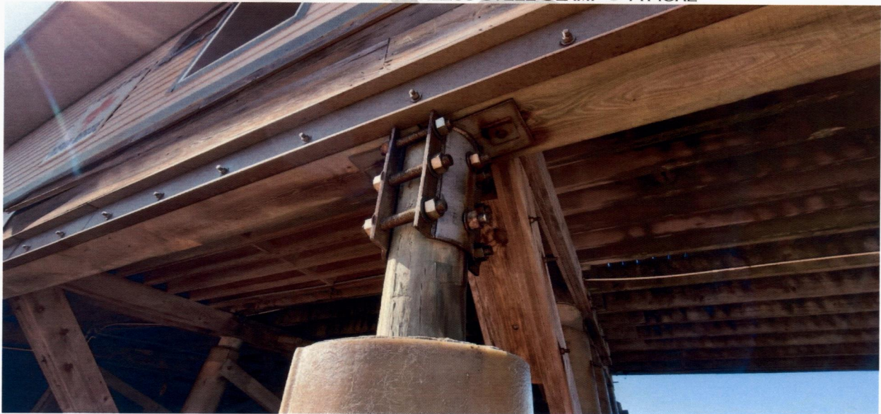
BENT 48 PILE J WITH STAINLESS STEEL CLAMP — TYPICAL
