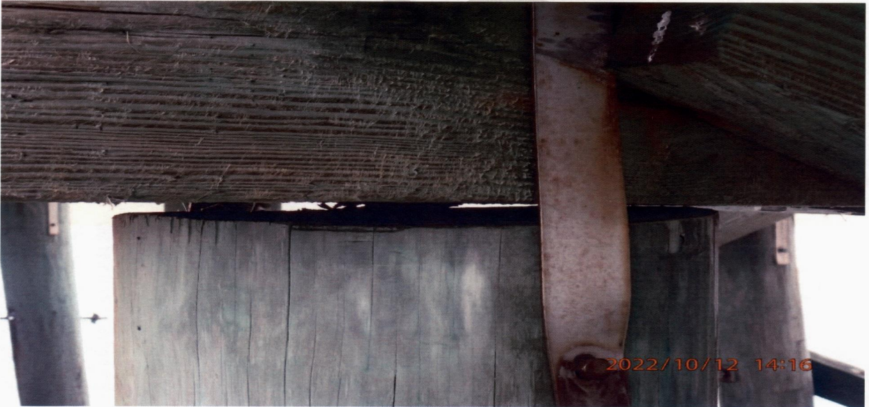
PILE 100% NOT TOUCHING THE CAP – TYPICAL
