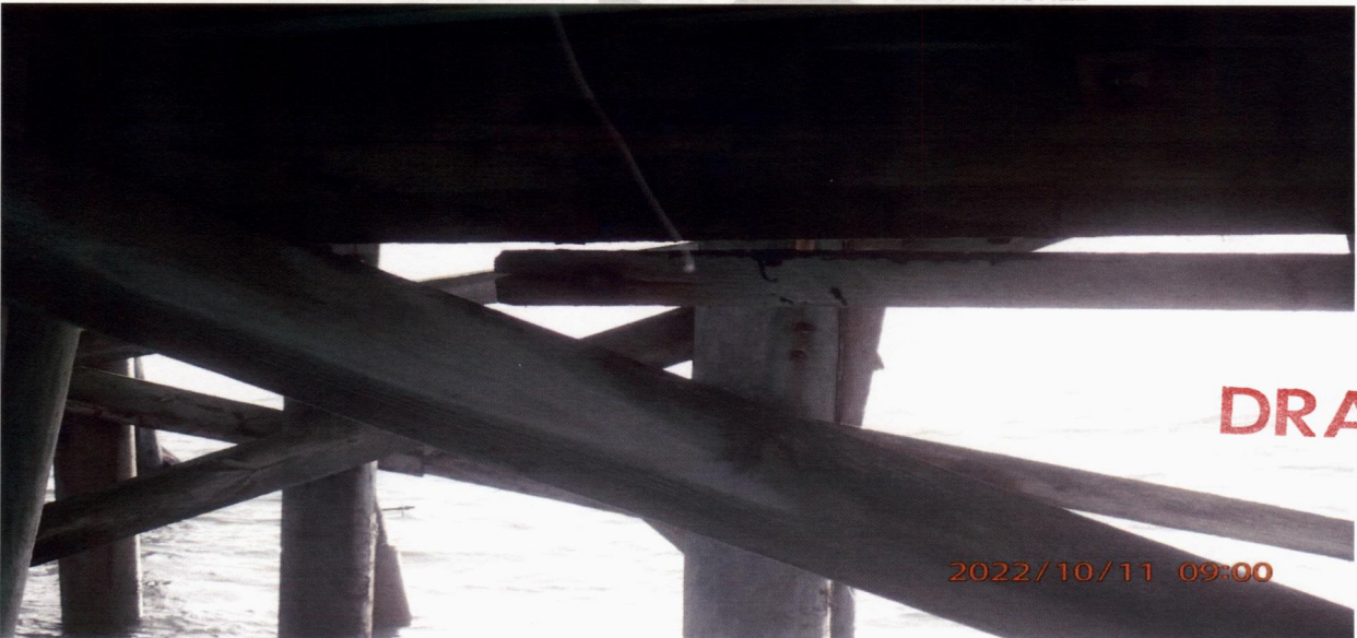
BENT 37 HORIZONTAL CROSS BRACE NO LONGER ATTACHED
