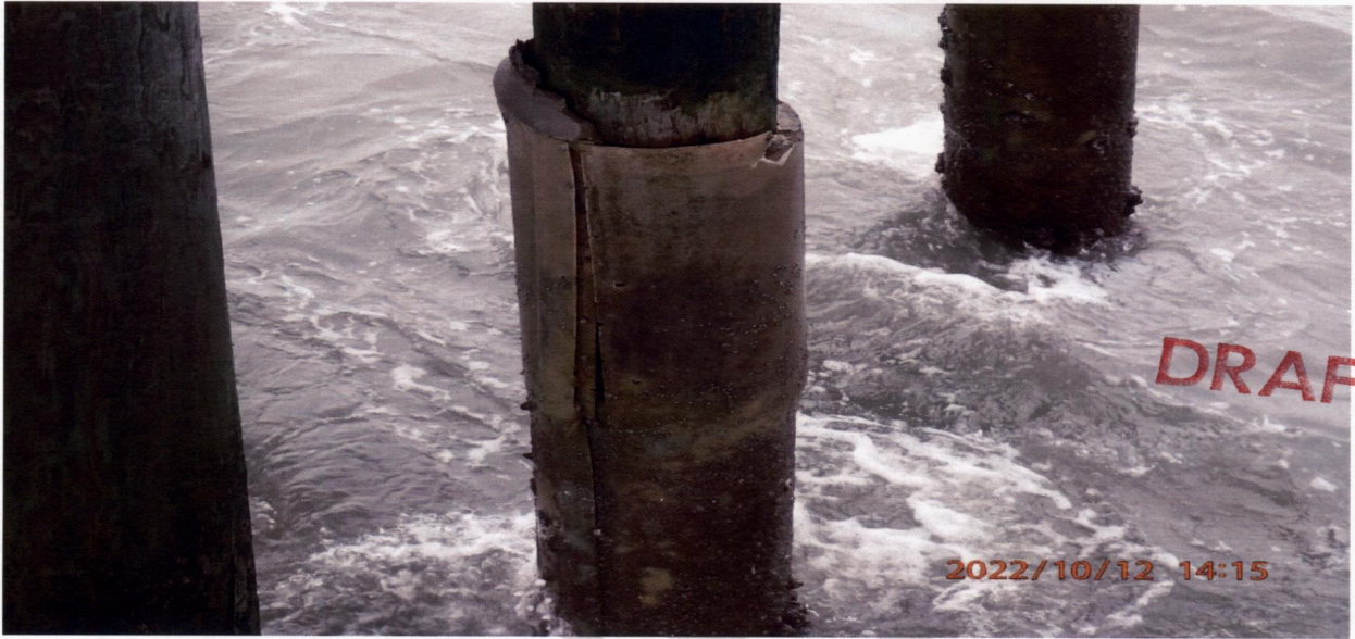
PILE 100% NOT TOUCHING THE CAP – TYPICAL
