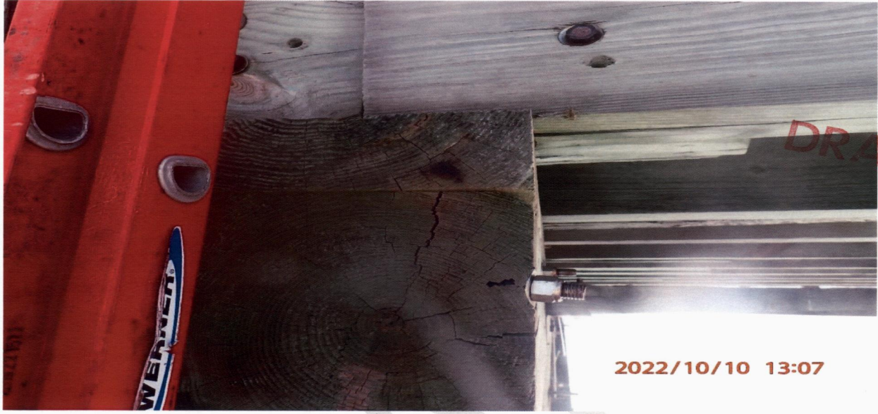
EXPOSED HOLLOWED PILE STUB ABOVE GL – TYPICAL
