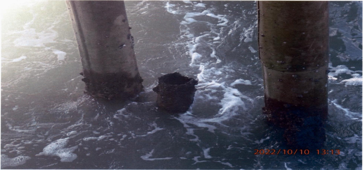
EXPOSED HOLLOWED PILE STUB ABOVE GL – TYPICAL
