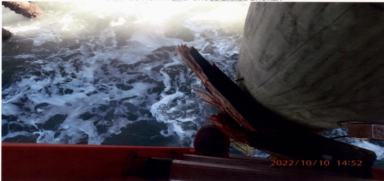
BENT 38 NORTH V/D CROSS BRACE BROKEN
