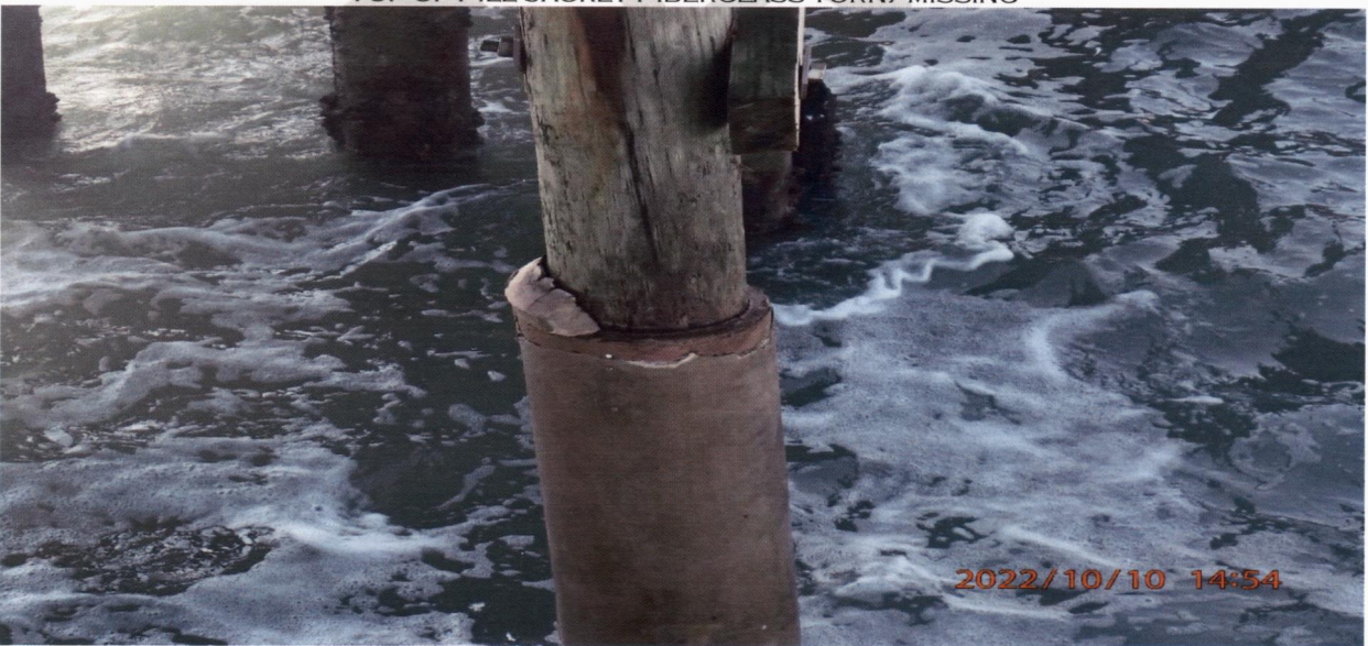
TOP EPOXY SEALS ON EVERY PILE JACKET ARE BROKEN/ CRACKED/ MISSING/ FAILED — TYPICAL TOP OF PILE JACKET FIBERGLASS TORN/MISSING
