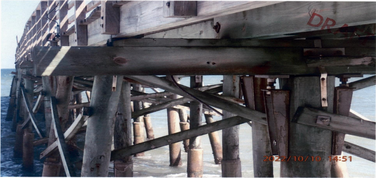
TOP EPOXY SEALS ON EVERY PILE JACKET ARE BROKEN/ CRACKED/ MISSING/ FAILED — TYPICAL TOP OF PILE JACKET FIBERGLASS TORN/MISSING
