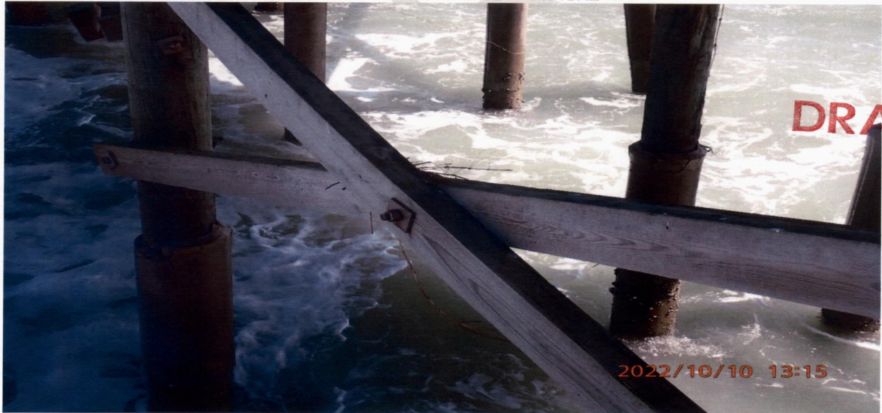
SOUTH CROSS BRACING – TYPICAL
