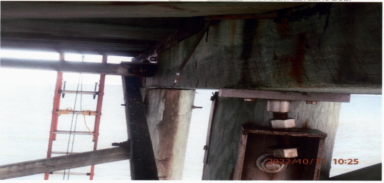
BENT 35 PILE F FAILED STAINLESS STEEL HURRICANE STRAP/BENT LEVELING BOLT
