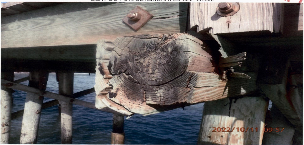
BENT 35 PILE F FAILED STAINLESS STEEL HURRICANE STRAP/BENT LEVELING BOLT
