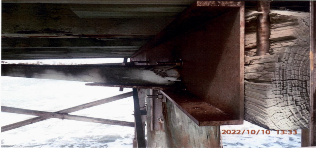
BENT 39 CAP REPAIR EASTSIDE
