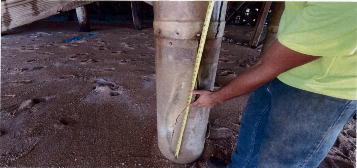
BENT 49 PILE F 5'x3" DEEP CRACK
