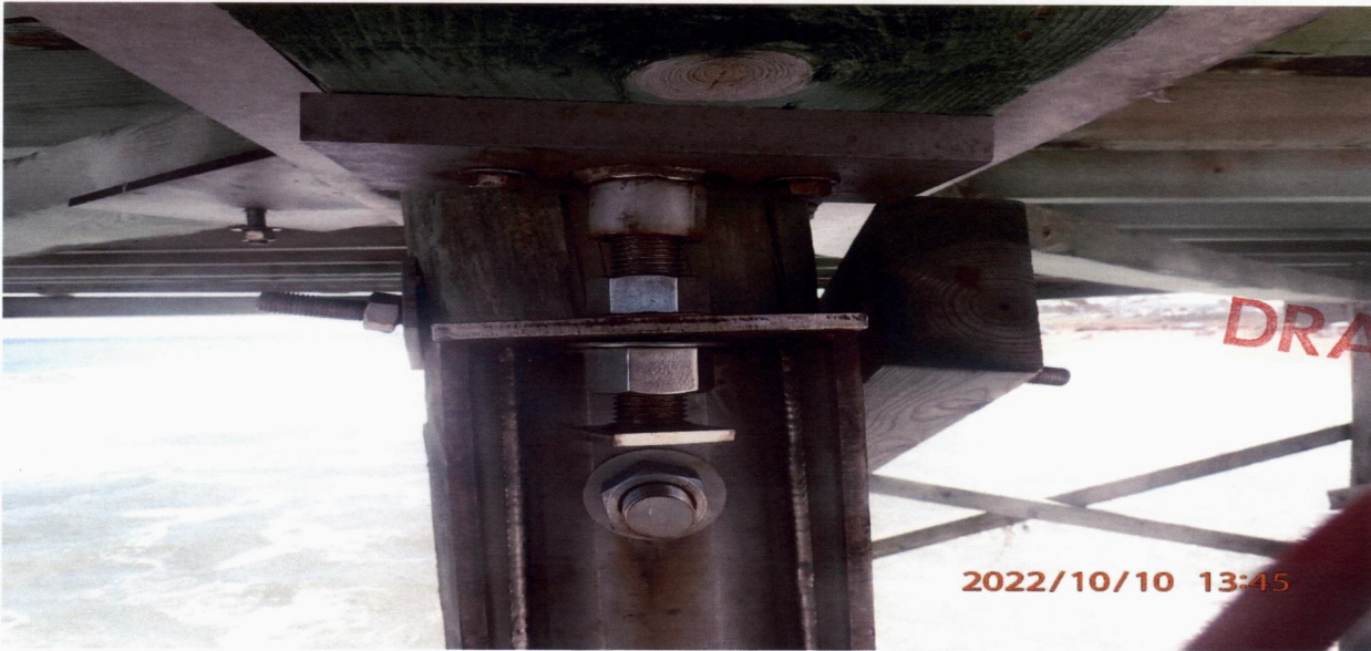
BENT 38 NORTH V/D CROSS BRACE BROKEN
