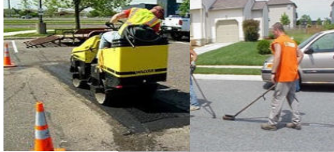
Patching/Crack Sealing
