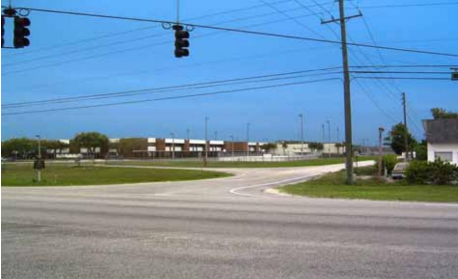
State Road 100/Bulldog Drive Intersection Facing North – Existing Condition
