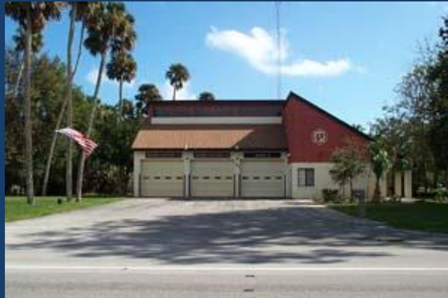
Palm Coast Emergency Services Building a.k.a Station #22
