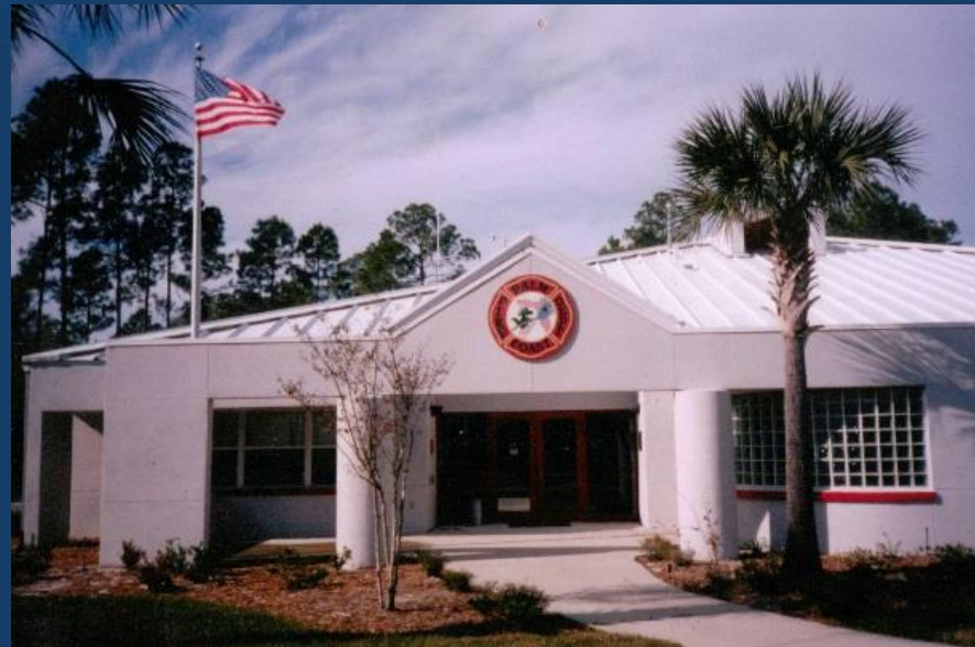
Palm Coast Opens 2 nd Fire Station a.k.a Station # 21
