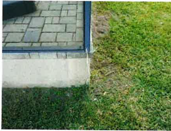
Photo 12-8 EXPOSED WIRES
