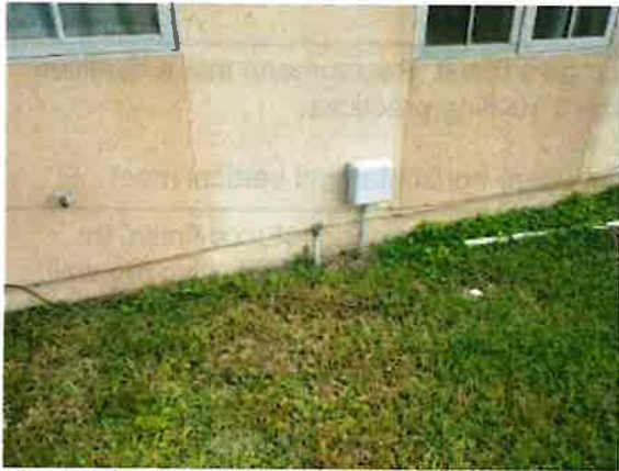
Photo 11-3 STUCCO REPAIR UNDER WINDOWS
