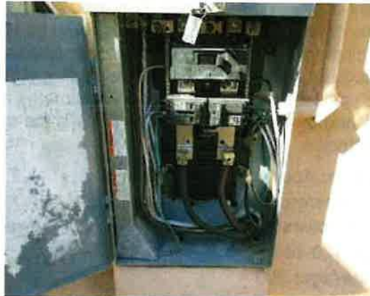
Photo 22-2 MAIN PANEL 200A FEED THRU
