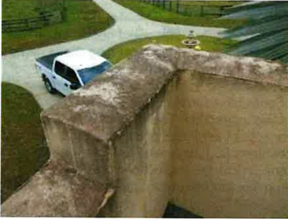
Photo 15-3 WALL MEETS TOP CAP STUCCO HAS OPEN JOINTS IN AREAS MAX 1/8 INCH
