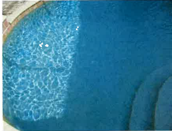
Photo 2-8 POOL SHELL REFER TO POOL REPORT
