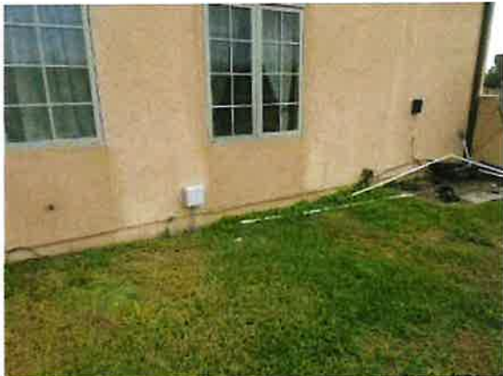
Photo 35-3 STUCCO REPAIR BELOW WINDOWS
