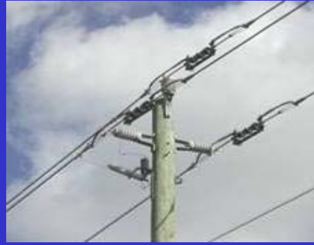
Feeder Switches
