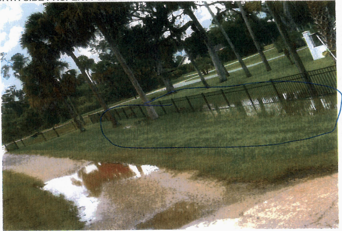
NORTH SIDE PROPERTY LINE after small rainfall
