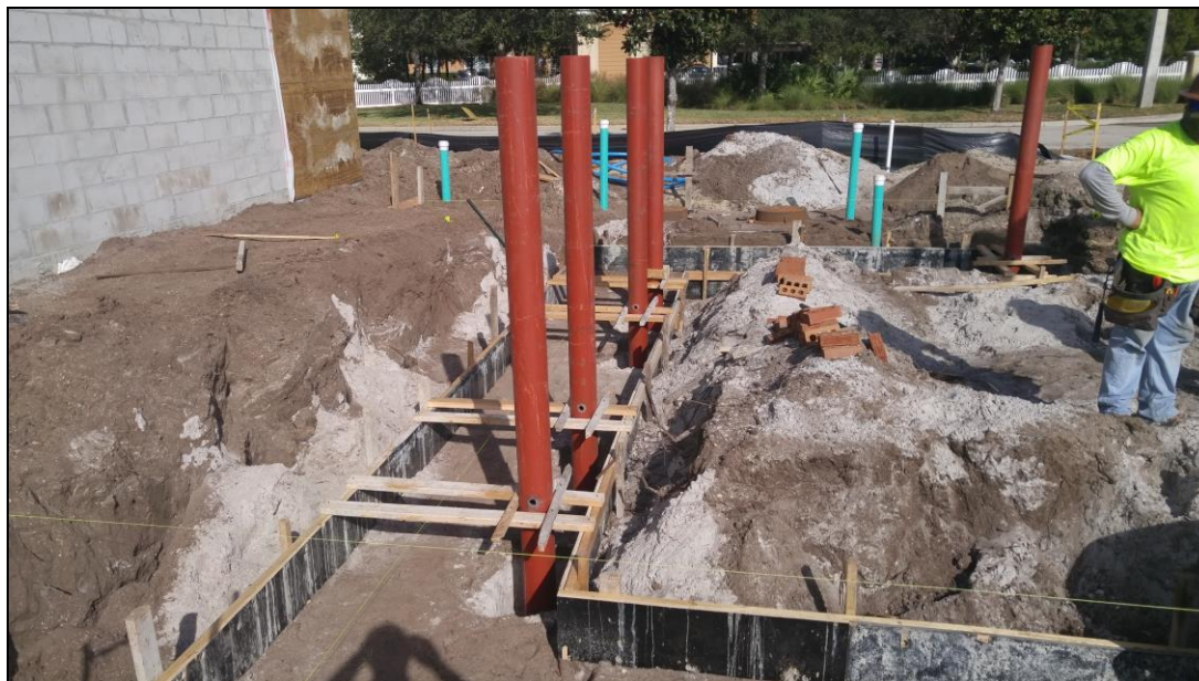
7-Eleven Store Form Boards for Dumpster Pad
