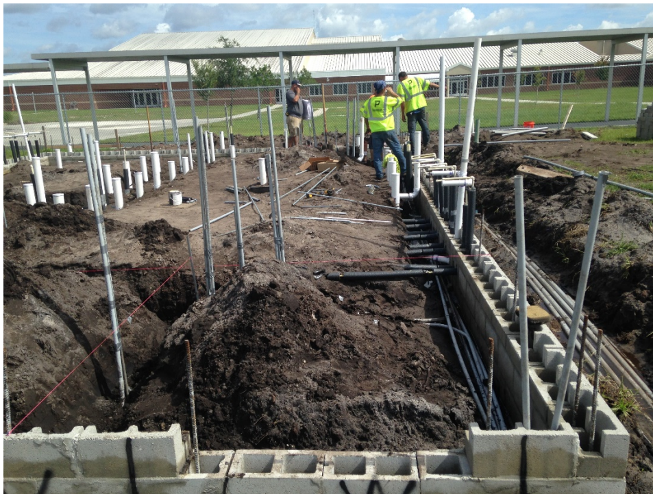
Indian Trails Sports Complex - Restroom Plumbing and Electrical
