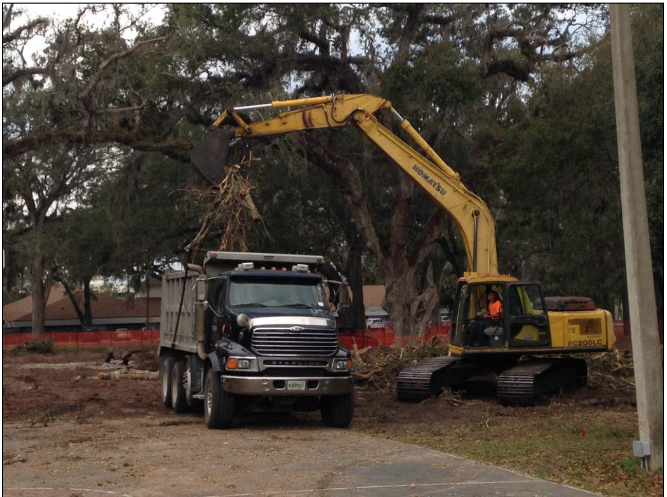
Demolished Trees Being Removed From Community Center Property
