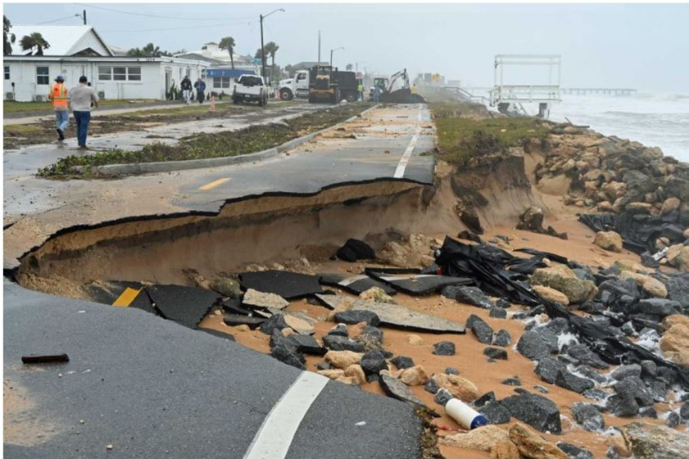
Several segments of State Road A1A in Flagler Beach and south of the city were carved out by waves unleashed by Tropical Storm Nicole, just three years after the Department of Transportation completed a $22.4 millio project to rebuild the road and add a sea wall further north. The sea wall held. The road did not. Two DOT contractors were already at work during the storm Thursday, dumping sand on breaches to stabilize what was left of the road. (© FlaglerLive)
