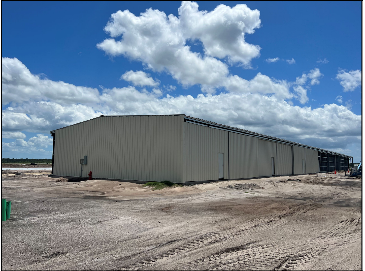
Construction completed on first building as of April 30, 2023
