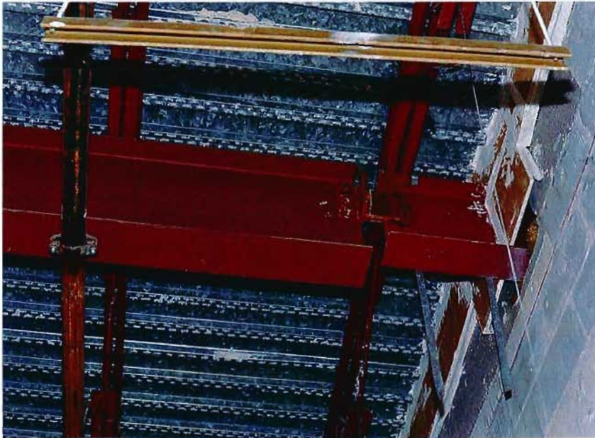
Beam Splice Connection of Dissimilar Beams
