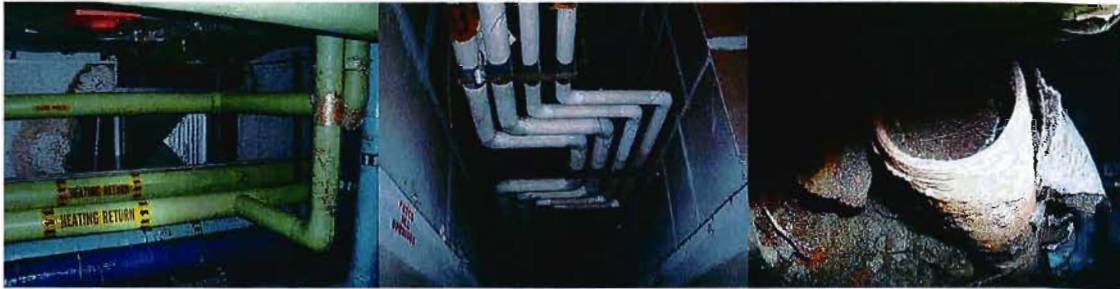
Typical Insulation and Pipe Conditions
