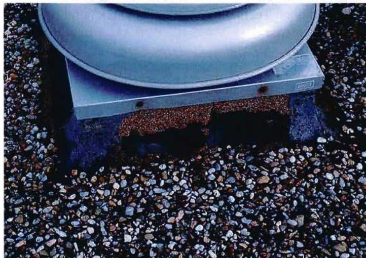
Built-Up Roof with Ballast
