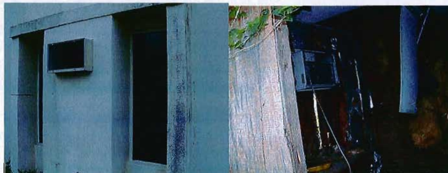
Condition of PTAC Units
