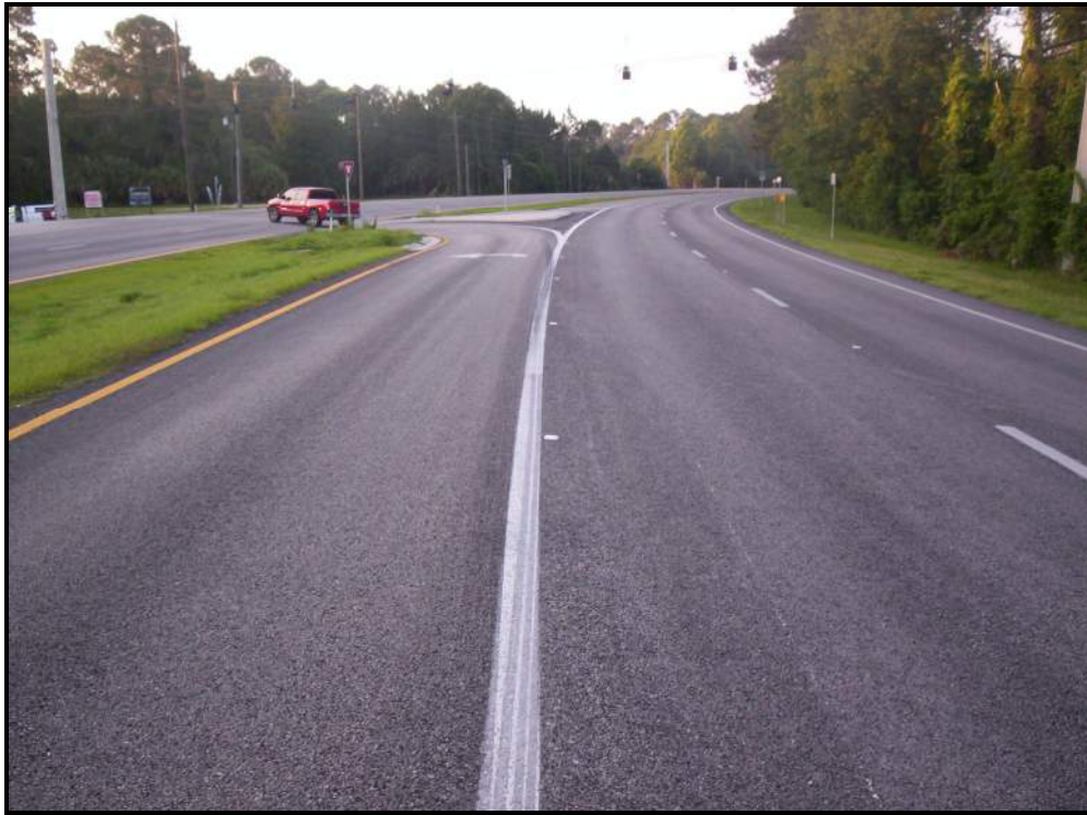
Looking south into the intersection along US 1
