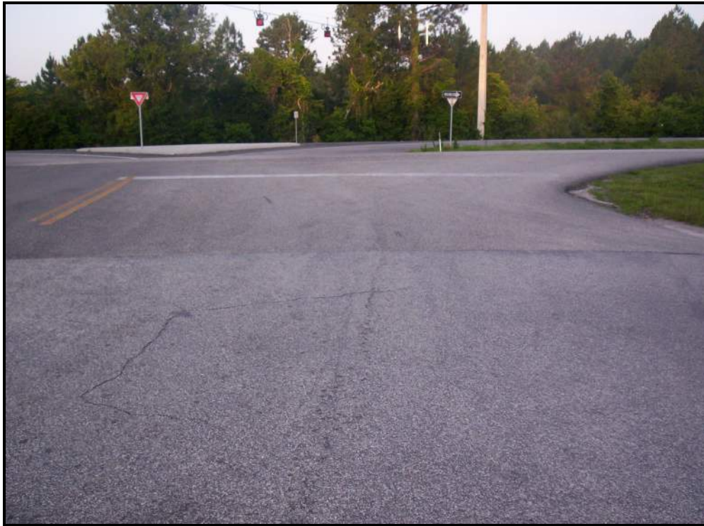
Looking east into the intersection along S Old Dixie Highway
