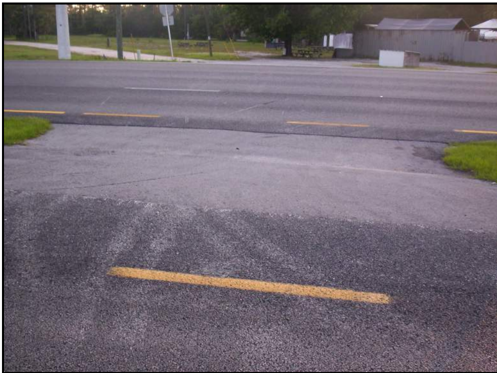
Looking east at the median from the west side of US 1
