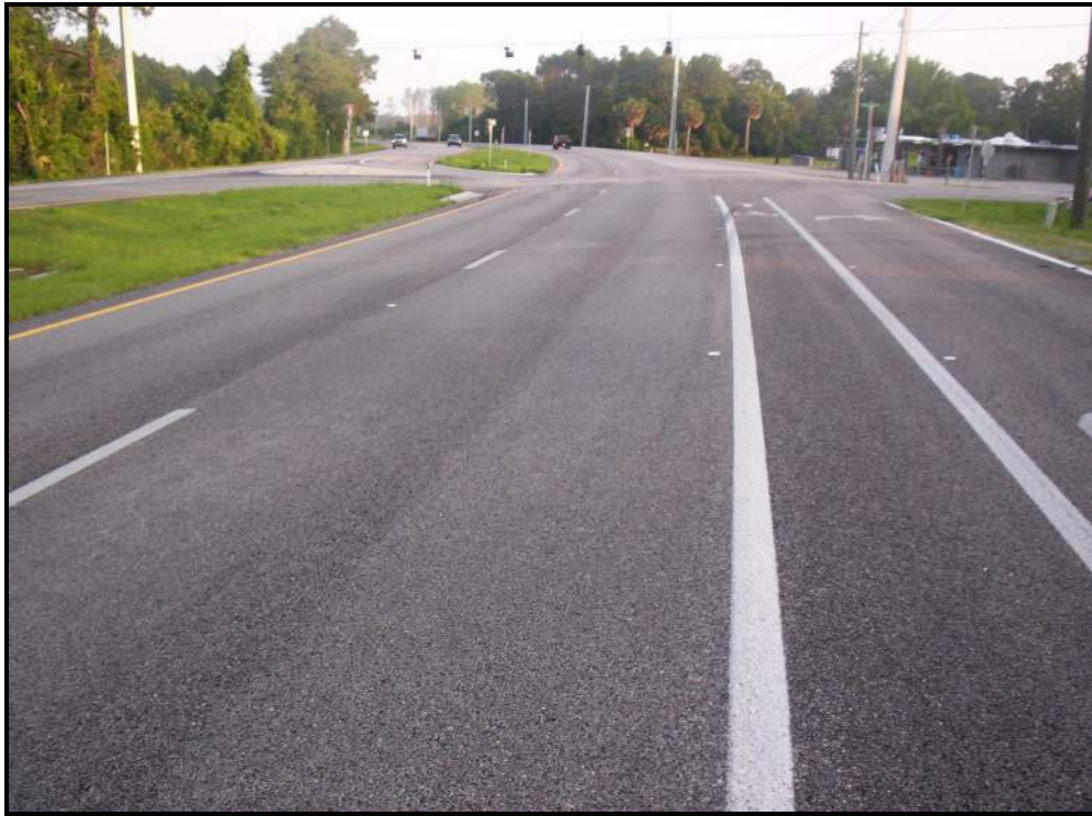
Looking north into the intersection along US 1
