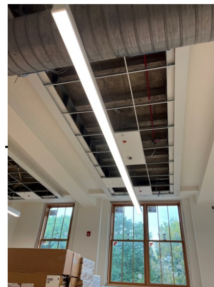
Above Ceiling Finish
