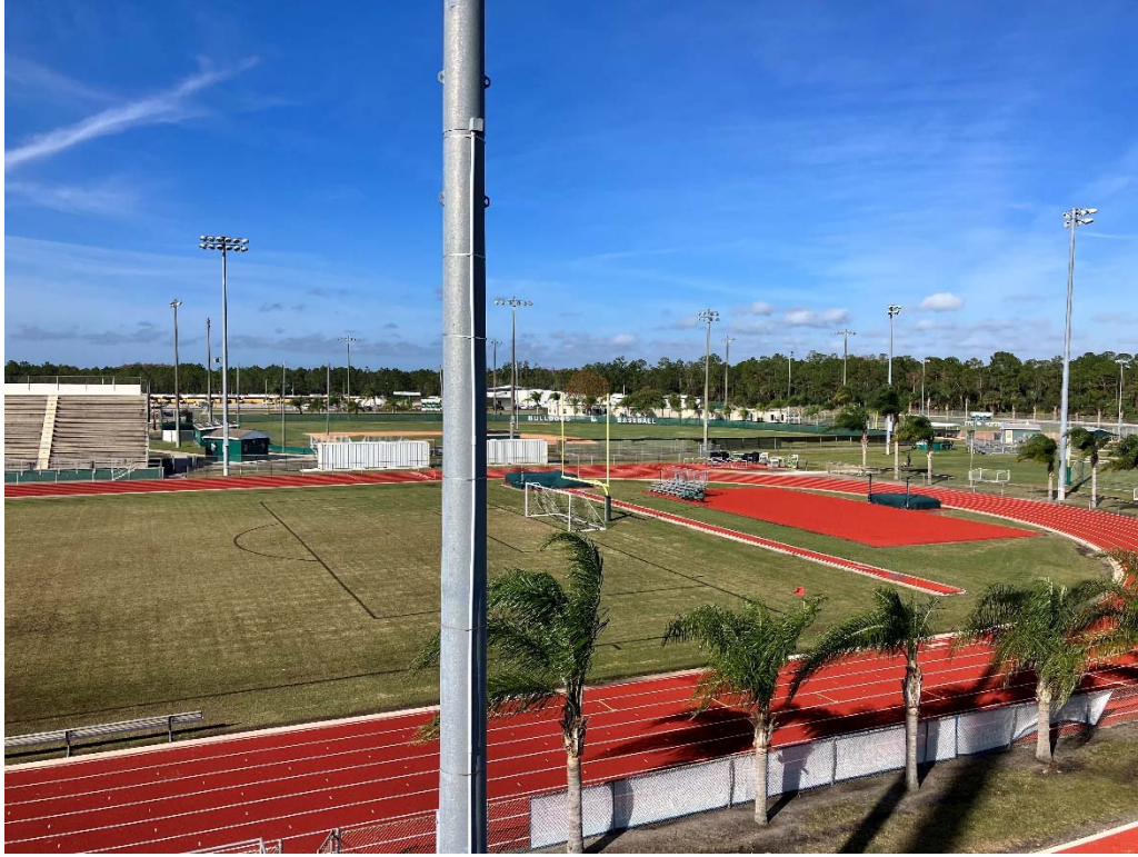
Figure 18: Site Photo – Photo from Bleachers facing Northwest
