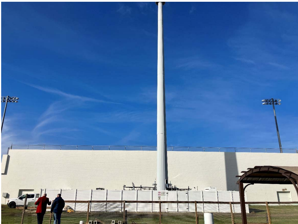
Figure 7: Site Photo - Equipment Compound East facing West
