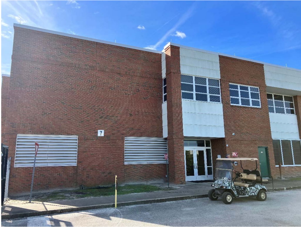
Figure 12: Site Photo – Building 7
