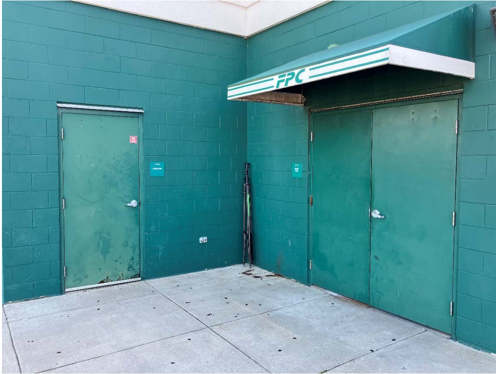
Figure 14: Site Photo – Building 12
