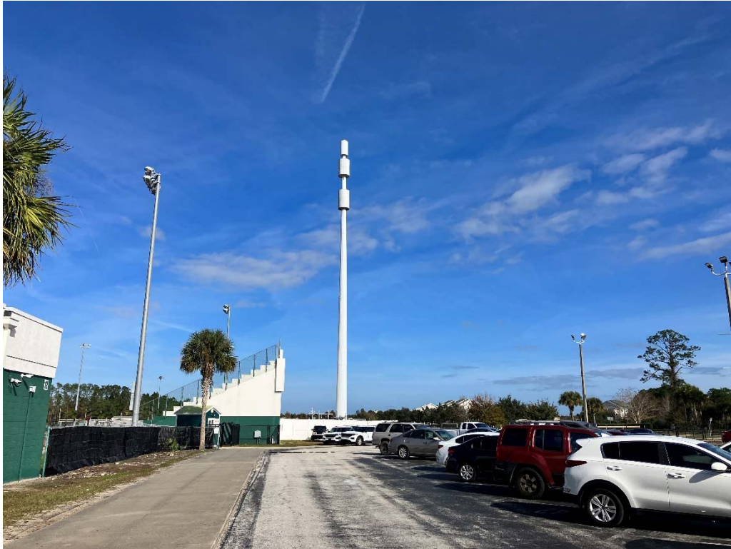
Figure 2: Site Photo – South facing North
