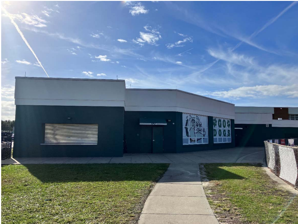
Figure 15: Site Photo – Building 12 Overview
