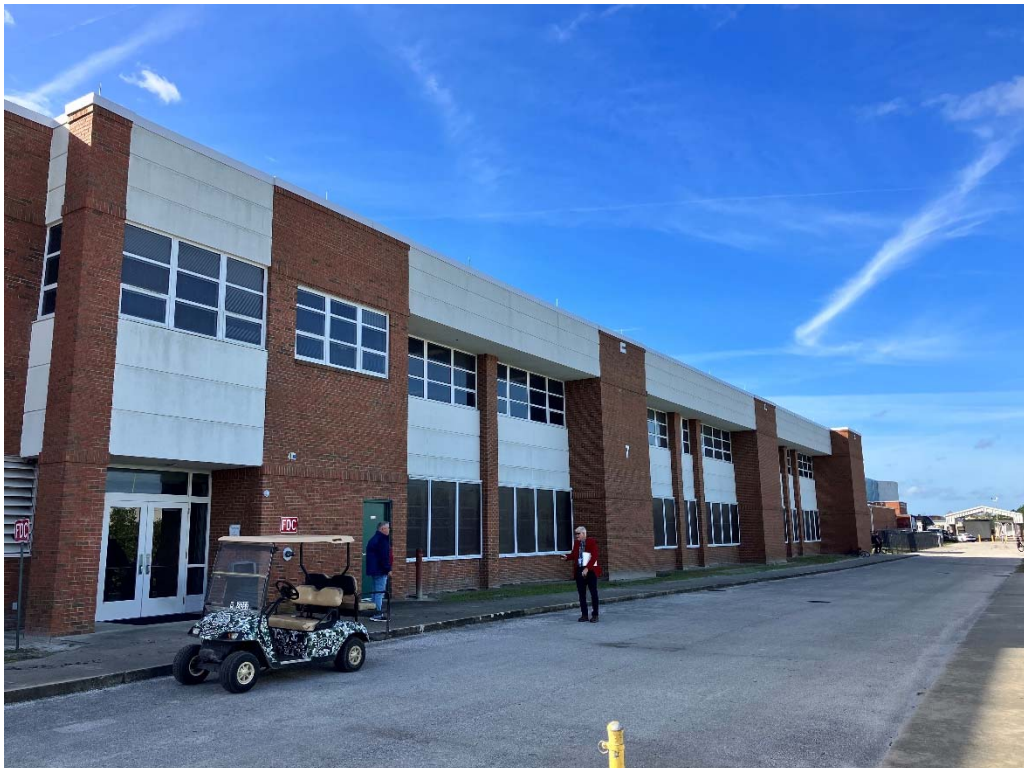
Figure 13: Site Photo – Building 7 Overview
