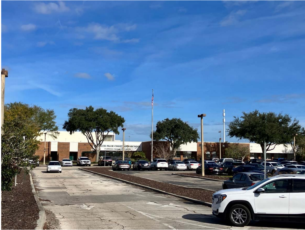
Figure 4: Site Photo – School Overview
