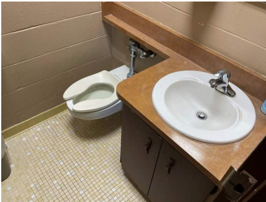
IMG_4354: Toilet and Lavatory
