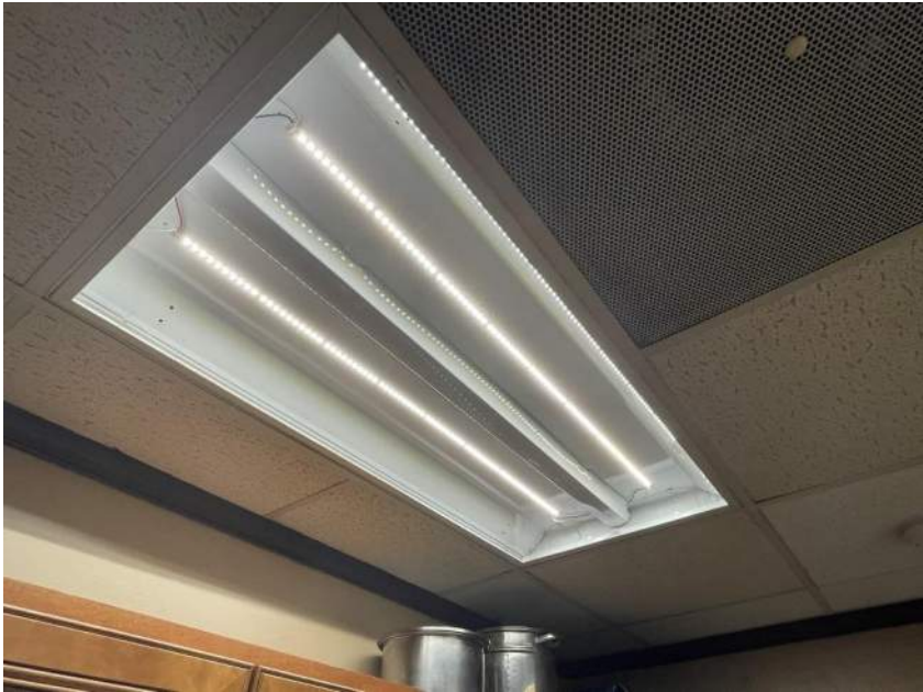
IMG_4378: LED retrofit of original light fixture
