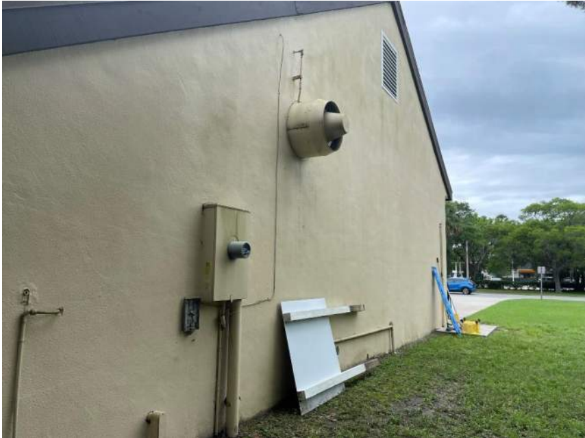
IMG_4326: Abandoned fan on east wall
