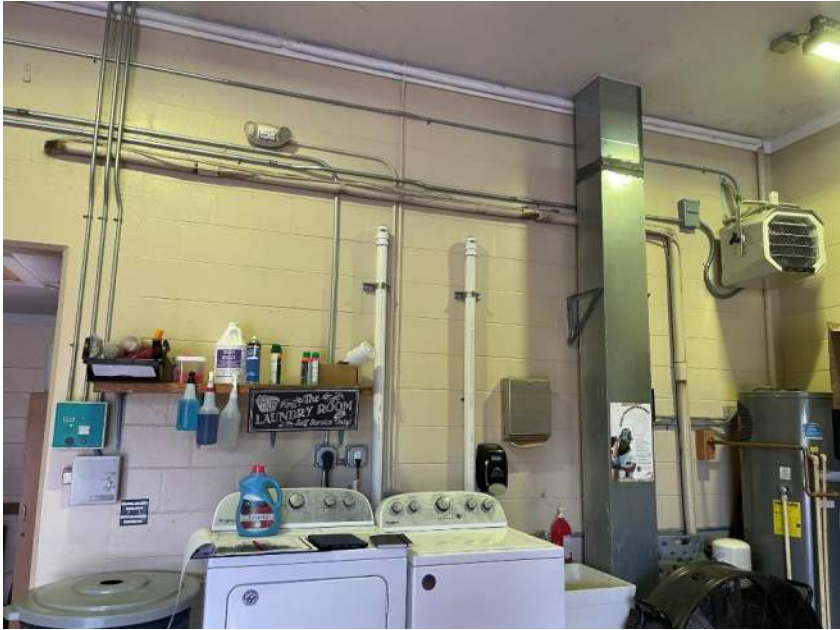
IMG_4301: Added emergency light
