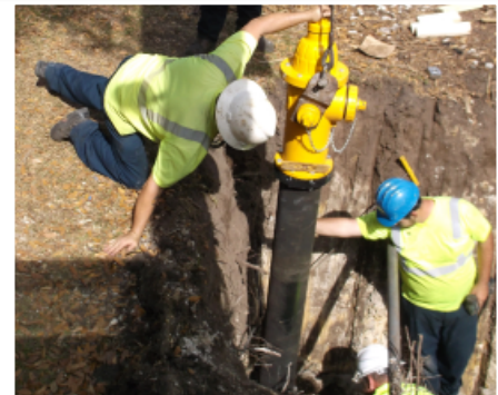
Installing New Fire Hydrant
