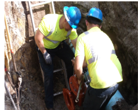
Installing New Fire Hydrant
