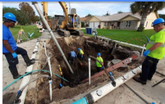
Gravity Sewer Main Repair
