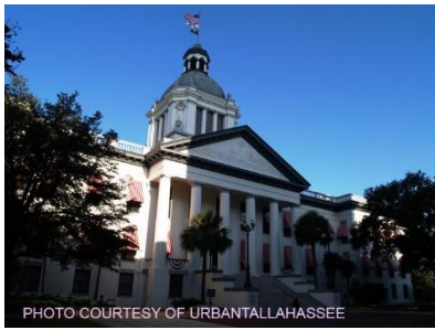
PHOTO COURTESY OF URBANTALLAHASSEE
