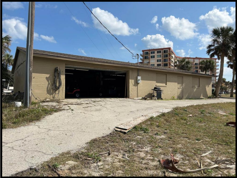
VIEW OF STORAGE BUILDING
