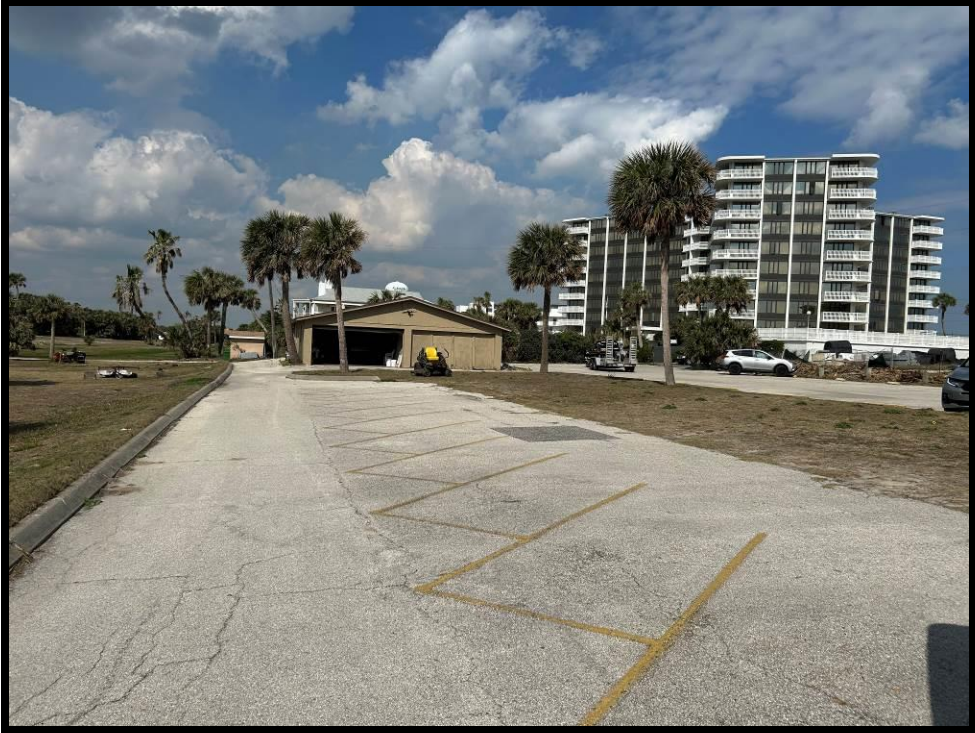
VIEW OF PARKING AREA
