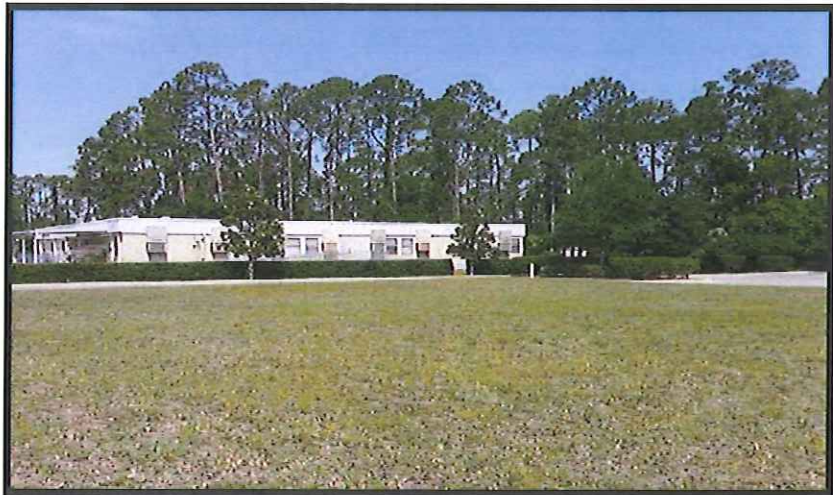
VIEW OF PORTABLE BUILDING FROM ADJACENT KOHL'S PARKING LOT
