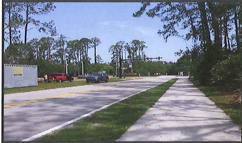
VIEW NORTH ALONG SITE'S CORPORATE DRIVE FRONTAGE
