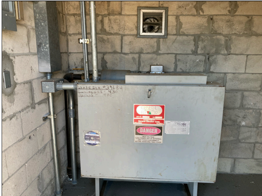
21 - Elevator room on roof of three-story building.
