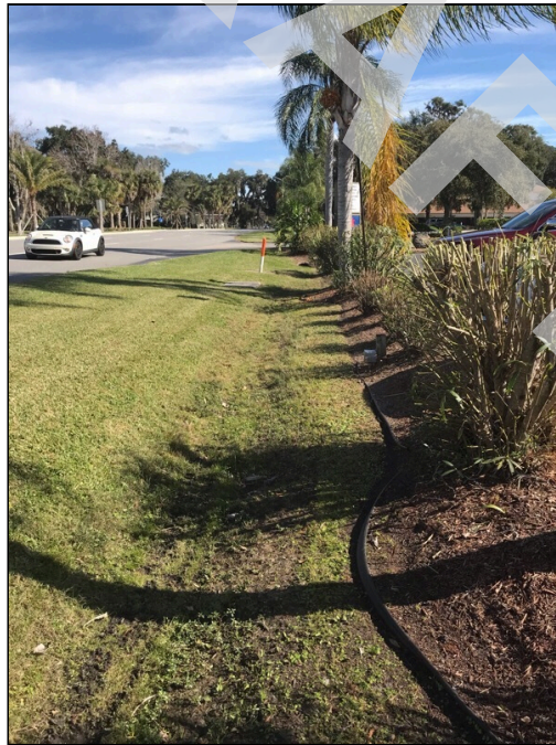
2 - Drainage ditch along the northern property boundary.
