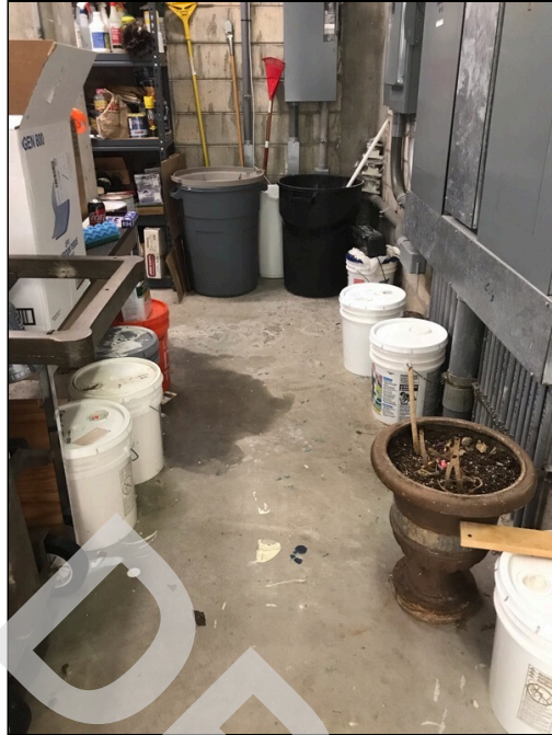
5 - First story supply room with paint buckets.
