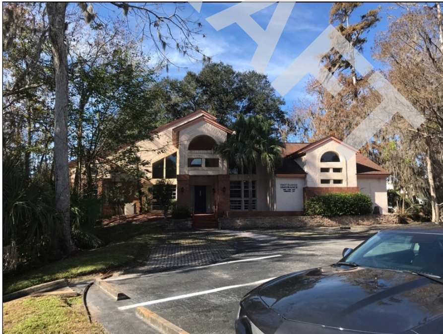
14 - Single-story office building on the southwest corner of the site.
