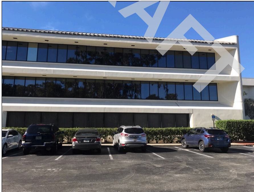
16 - Eastern side of three-story office building.
