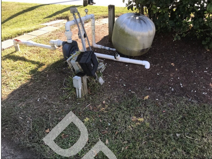
13 - Irrigation well on the southeast corner of the site.
