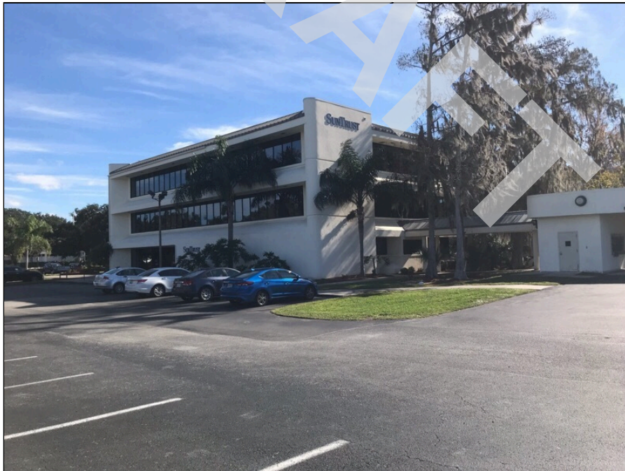
12 - Northern side of the three-story office building, facing southeast.
