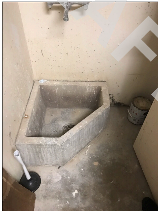
10 - Floor drain in a supply closet on the second floor of the three-story office building.
