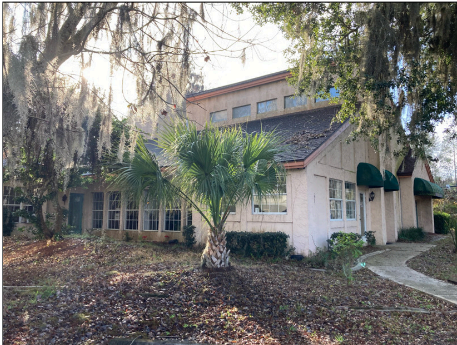
4 - Southwestern portion of subject property.
