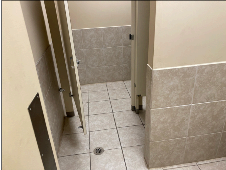
19 - Representative picture of bathrooms in the three-story building.
