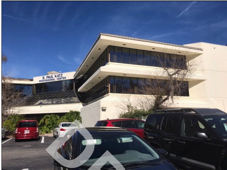
9 - Southern side of the three-story office building.
