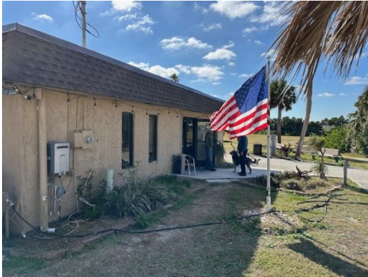
North side of the subject clubhouse
