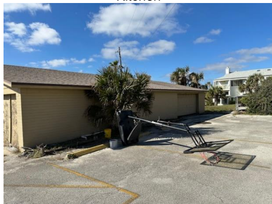
East side of the garage
