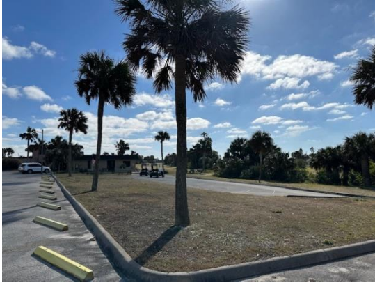
View of the subject property from the parking lot looking southwest
