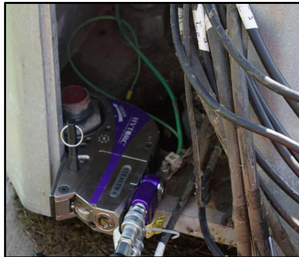
Figure 17-25: Recommended Hydraulic Torque Wrench
