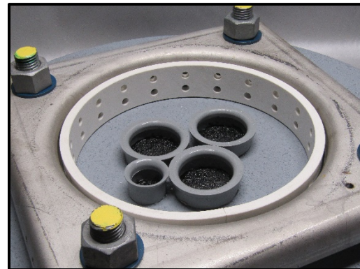
Figure 17-41: Approved Rodent Intrusion Barrier Found on MnDOT’s APL New Design to Fit Base Plate Change
