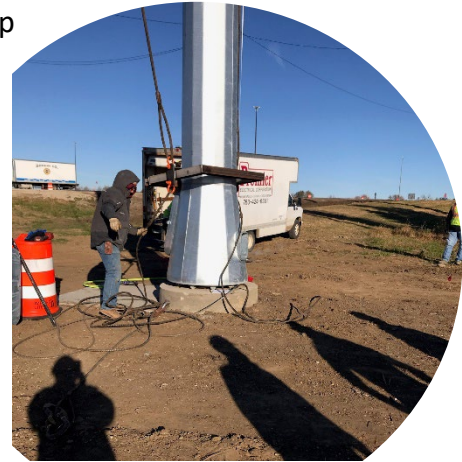
Figure 17-36: Setting a High Mast Light Tower with A Crane
