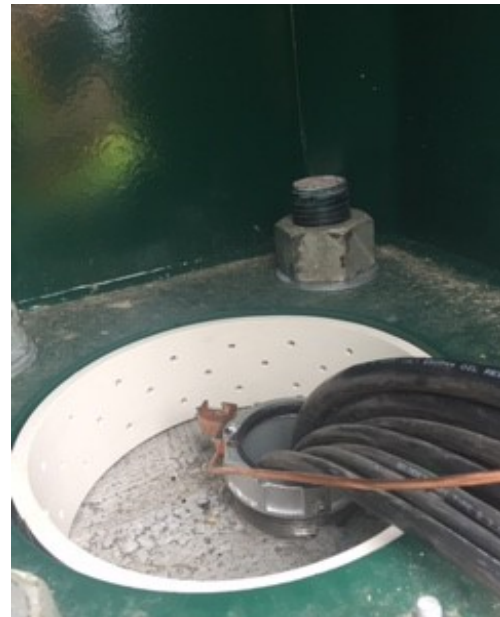
Figure 17-39: Approved Rodent Intrusion Barrier Found on MnDOT's APL
