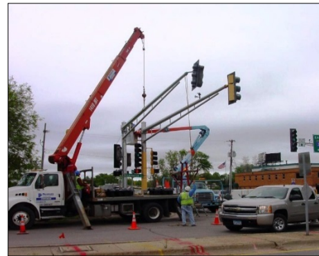
Figure 17-5: Signal Mast Arm Pole Installation
