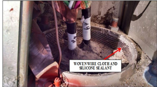
Figure 17-40: Woven Wire Cloth for Rodent Protection
