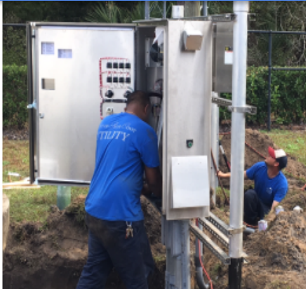
Pump Station Upgrades
