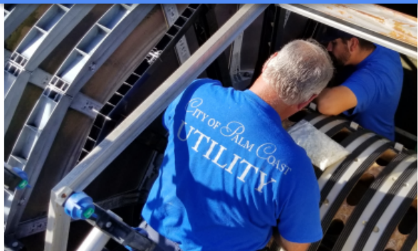
Installation of Filters
