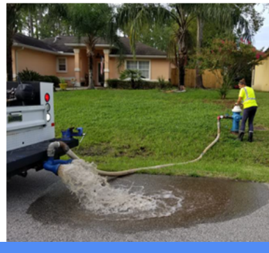
Unidirectional Flushing of Potable Water
