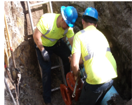
Installing New Fire Hydrant
