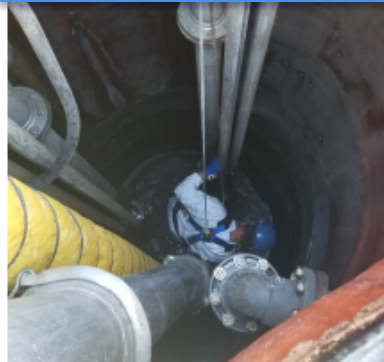
Evaluating Pump Station Pipes
