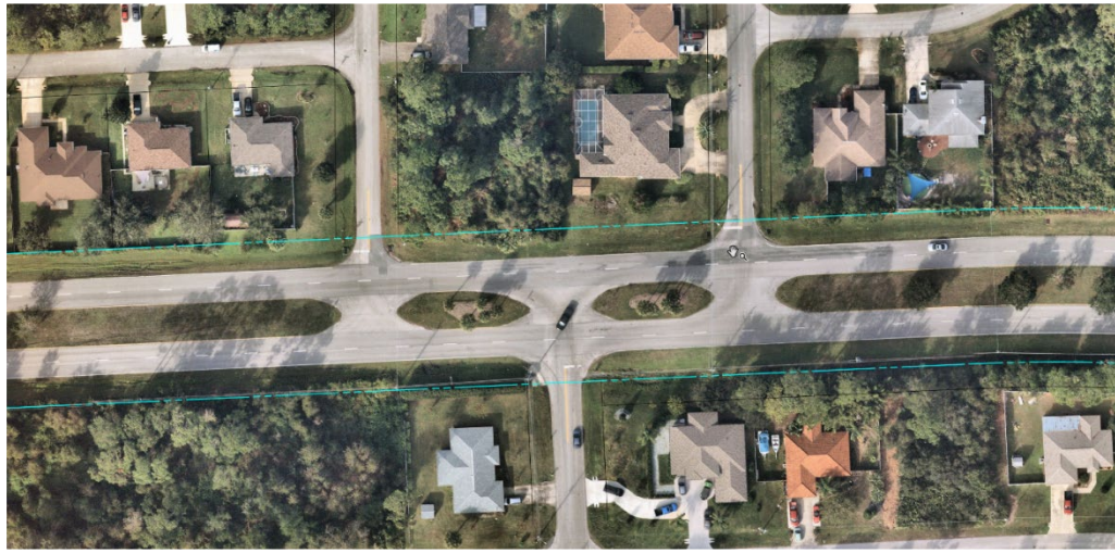
Rolling Sands Drive Existing Conditions
