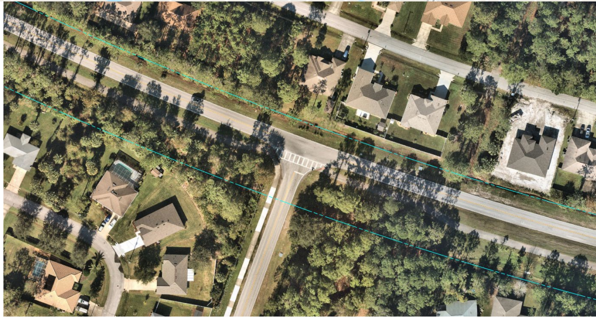
Ravenwood Drive Existing Conditions
