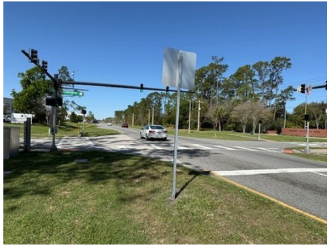
Intersection of Corporate Drive and Palm Coast Parkway NW
