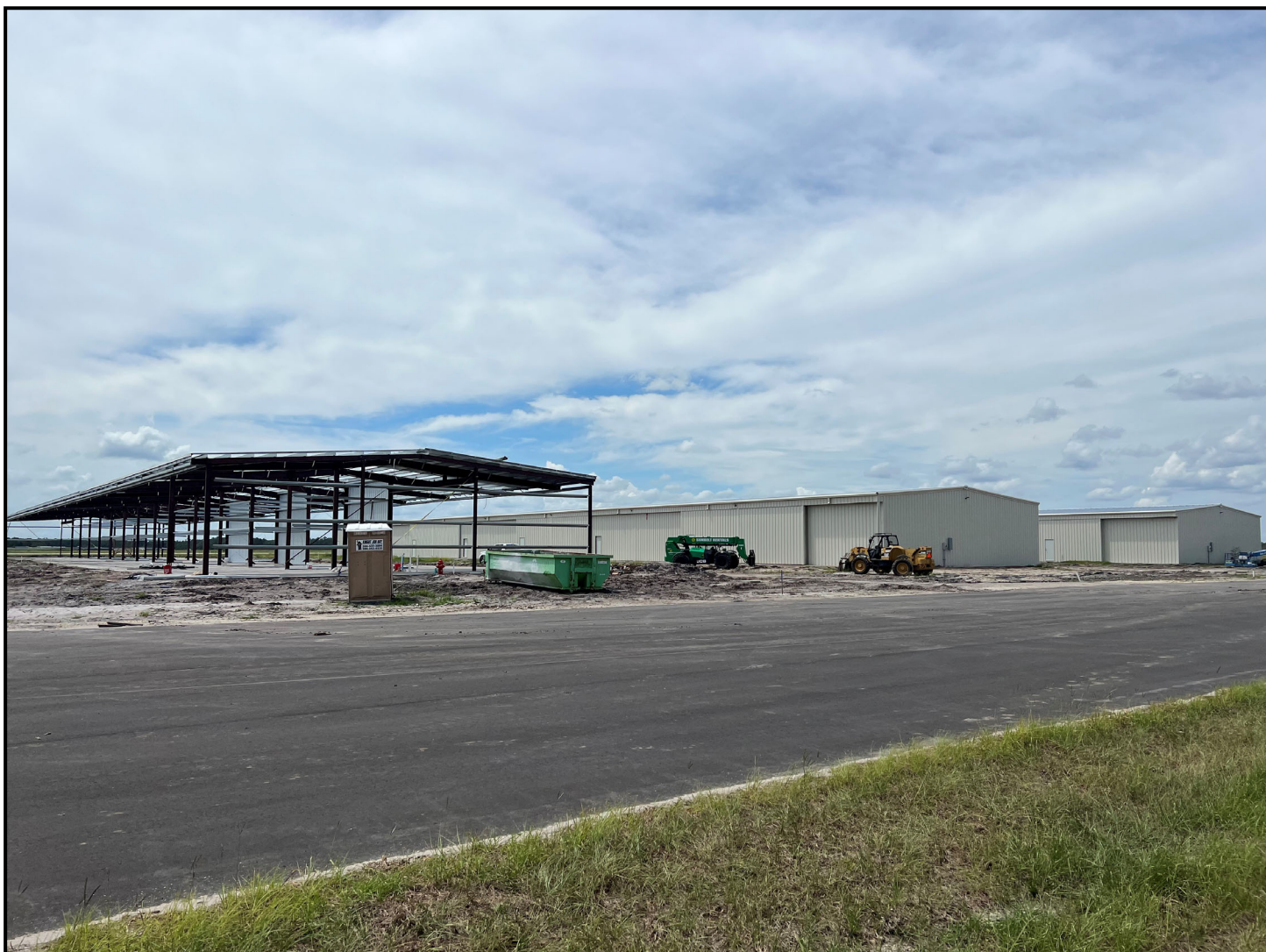
Construction completed as of August 29, 2023
