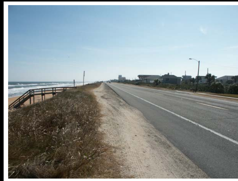
South Flagler Beach Existing Photo - Looking South
