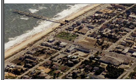
Existing Condition Of A1A - Through Flagler Beach
