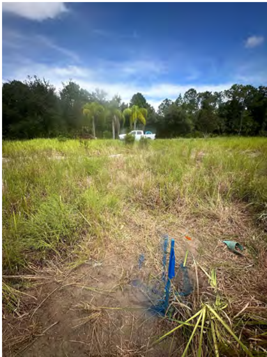
Photo No. 3 Site Image
