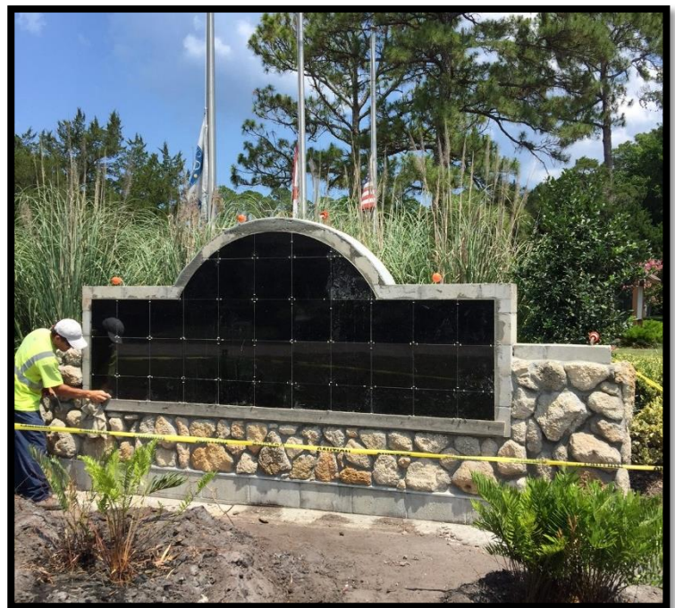
Tile Setting - Utility Administration Sign
