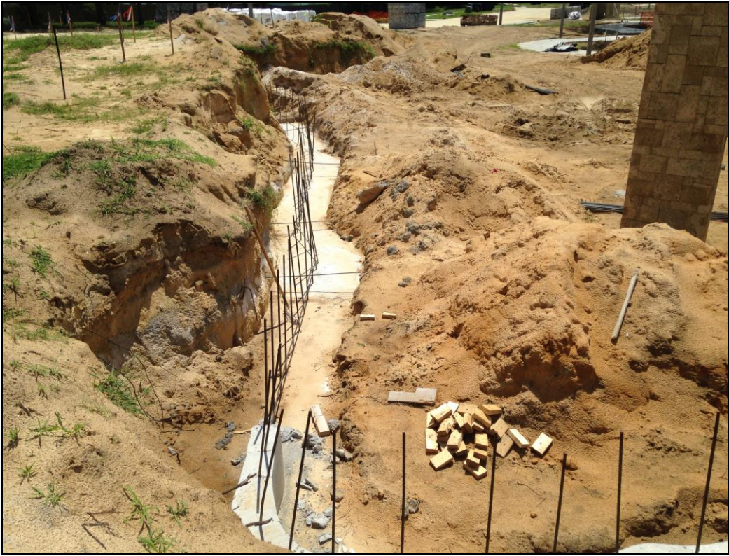
Lower Foundation for Playground Rock Wall
