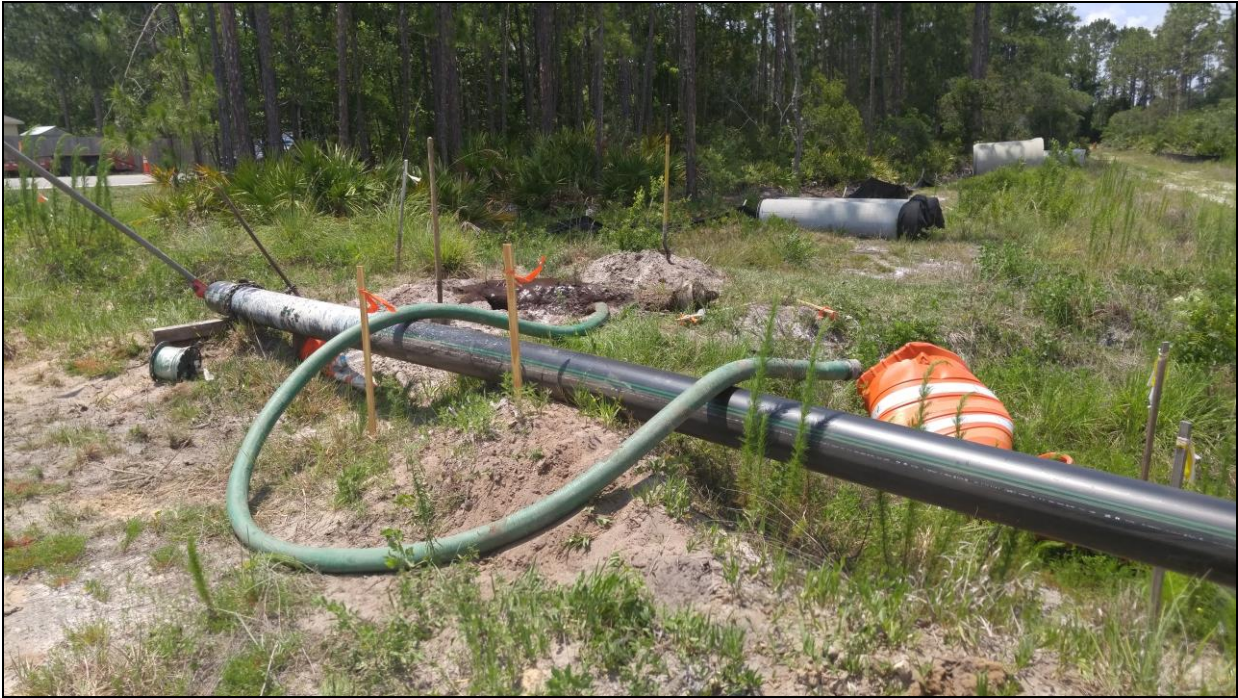
Airport Entrance 8' Force Main Directional
