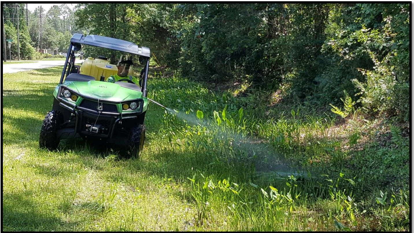
Drainage Ditch Herbicide Spraying
