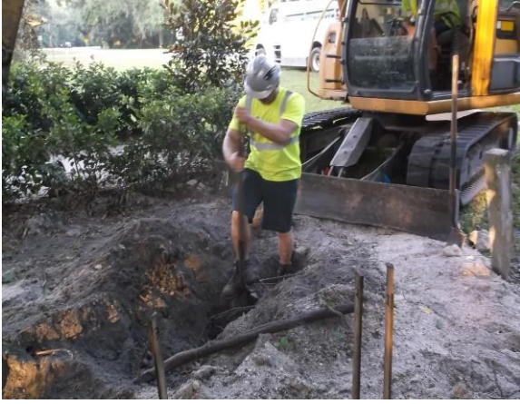
Lots of hand digging around existing utilities
