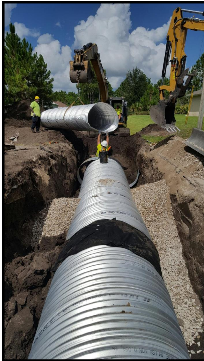
Stormwater Modeling - Pipe Replacement
