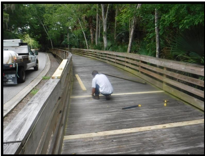
Pedestrian Bridge Repair Waterfront Park
