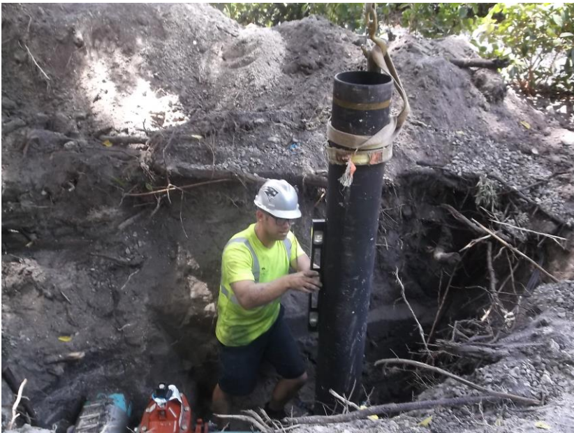
Plumbing the riser pipe that will connect to the new meter and backflow assembly
