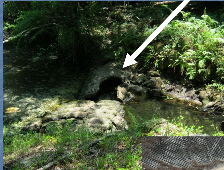
M-2 Structure Mulberry Creek Hazard Rating = 1
