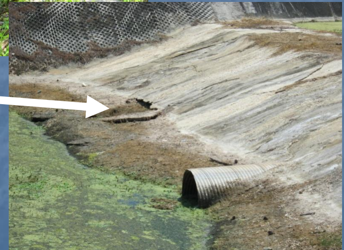
R-1 Structure Royal Palms Canal Hazard Rating = 6
