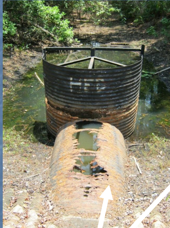
L-1 Structure Structural Rate = 6
