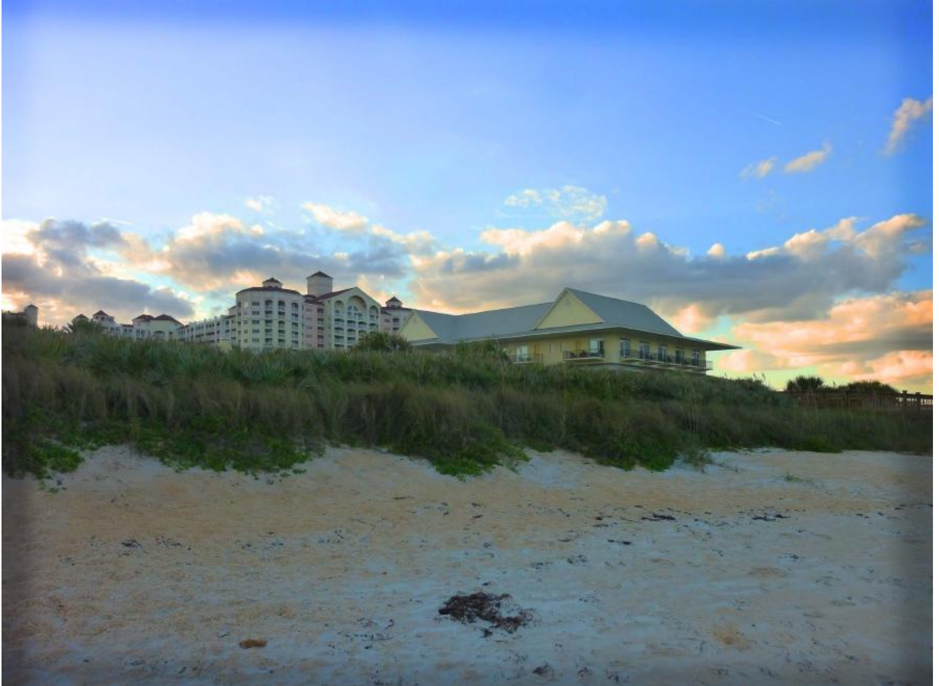
FIGURE 4A: VIEW OF PROPOSED CLUSTER 35 FROM BEACH (LODGE IN FOREGROUND, CLUB IN BACKGROUND)
