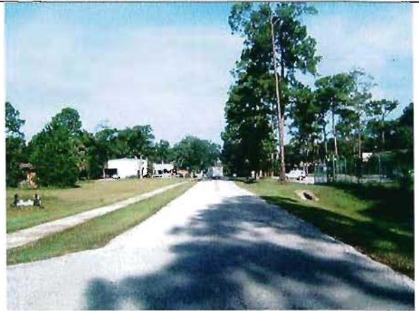
South Lemon Street Looking North; Improved Building Site Is To The Left.
