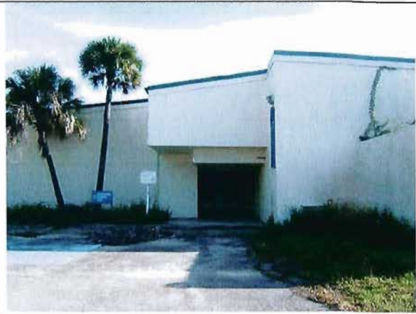
West Entrance To Former Emergency Department.
