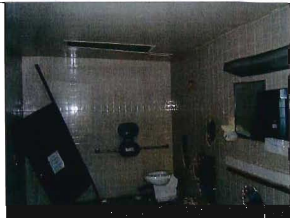
Typical Interior Room In Shell Condition.
