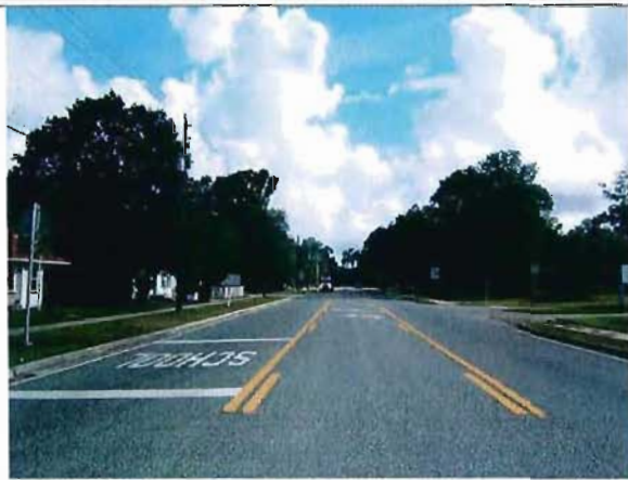
East Moody Boulevard (State Road 100) Looking East; Main Entrance To The Subject Is To The Right.
