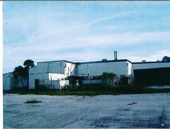
West Elevation Of Former Hospital Building.
