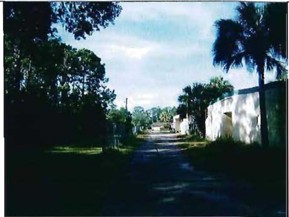
Rear Of Former Hospital Building Looking West Along The Rear Driveway.
