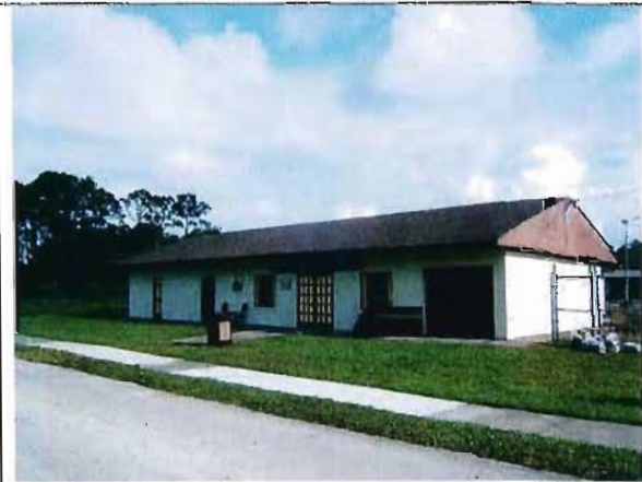
Maintenance/Storage Building Looking East Across South Chapel Street.
