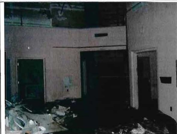
Typical Interior Room In Shell Condition.
