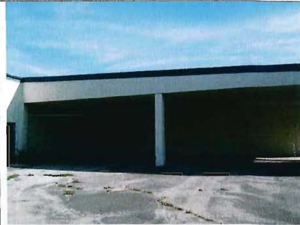
Former Covered Physician Parking.
