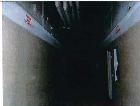
Interior Corridor Near Former Emergency Department; Typical Shell Condition.
