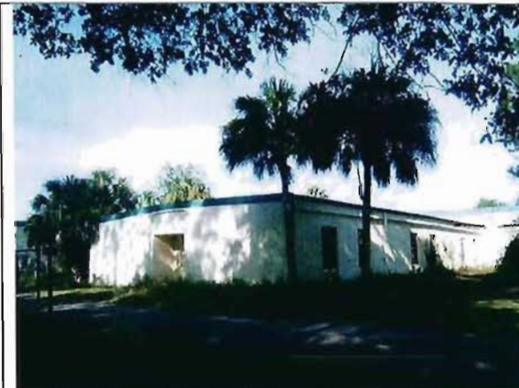
Former Patient Room Wings On The East End Of The Former Hospital Building.
