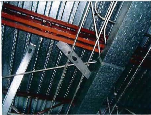
Roof Structure With Steel Trusses And Metal Decking.
