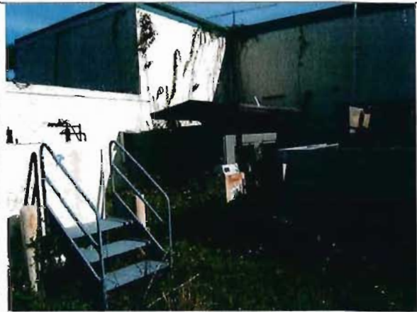
Emergency Generator In The Background; Concrete-Vaulted Fuel Storage Tank To The Left.
