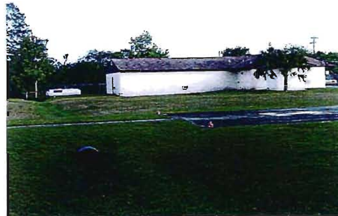
Hospital maintenance facility
