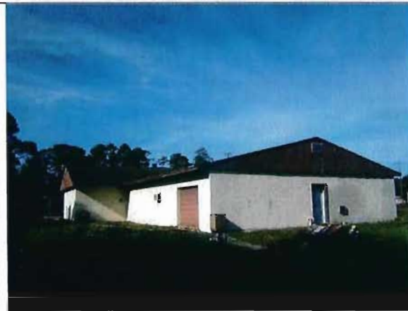
Maintenance/Storage Building Looking West From Near Former Hospital Building.
