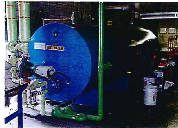
Hot water tank
