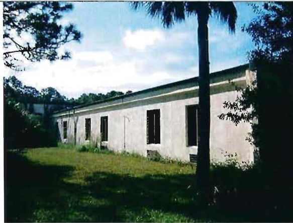
Former Patient Room Wings On The East End Of The Former Hospital Building.
