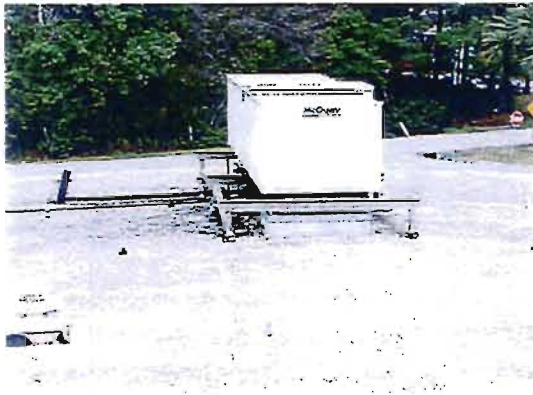
Roof AHU
