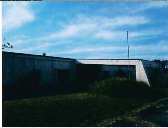
Front Entrance To The Former Hospital Building Looking South From Near Canakaris Street.
