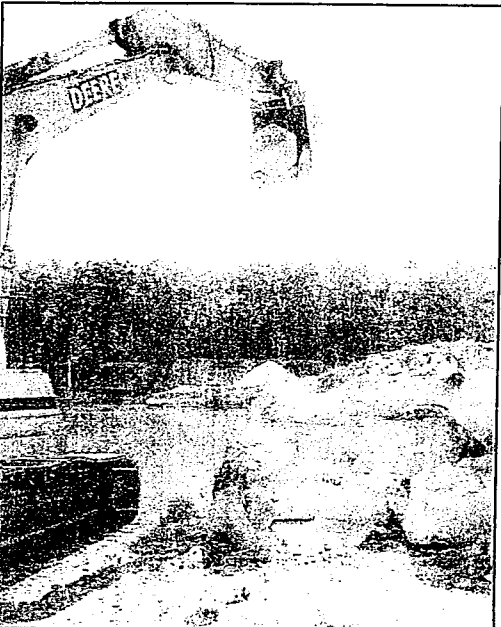
John Deere 350D track excavator dropping specially constructed wrecking "ball" for breaking apart
